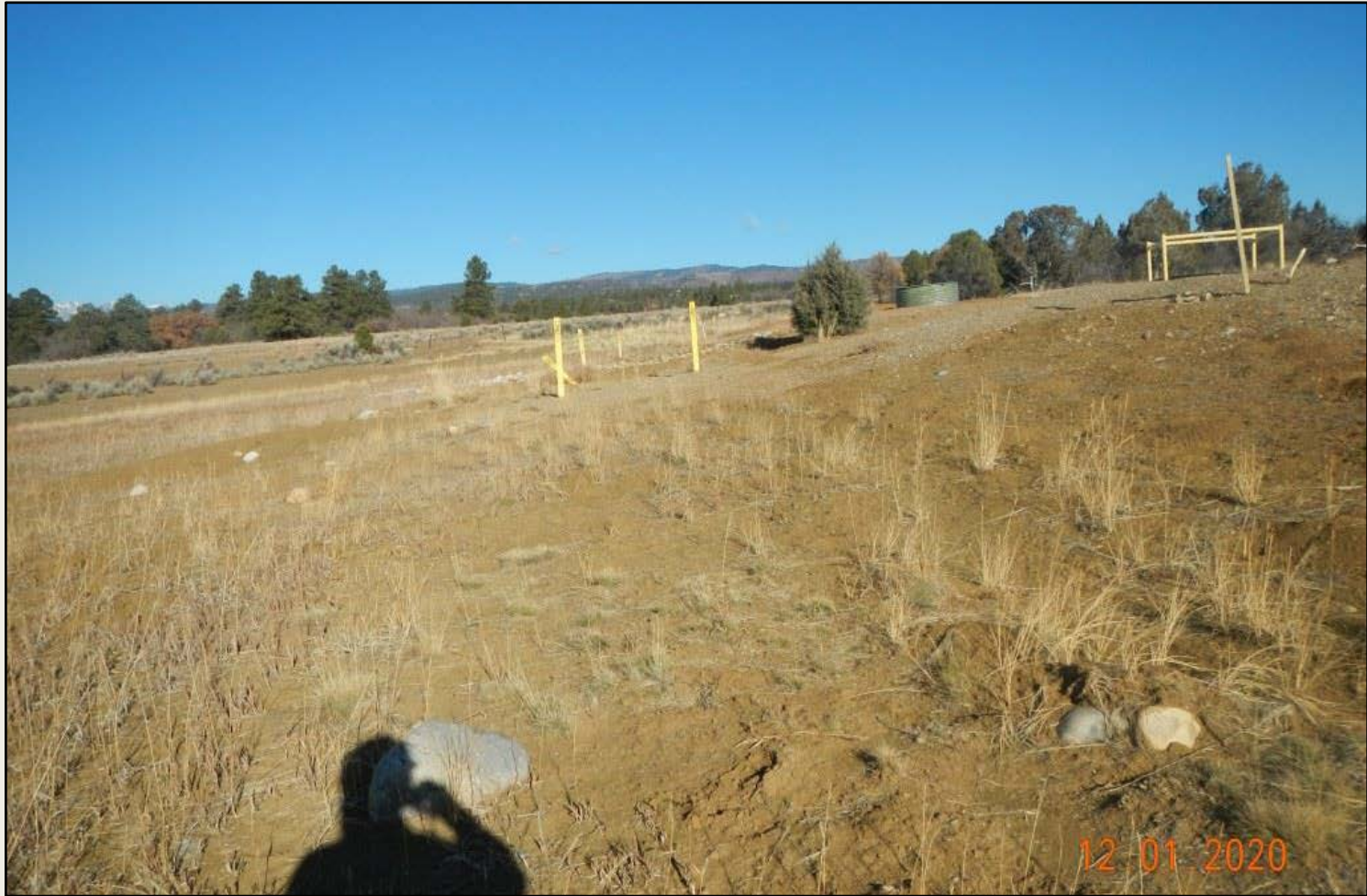
Photo 4. View of the western project area from the southwestern corner facing northward. Gravel and cobble placed where water flows off of the well pad. This will need to be monitored and maintained when erosion occurs here.
