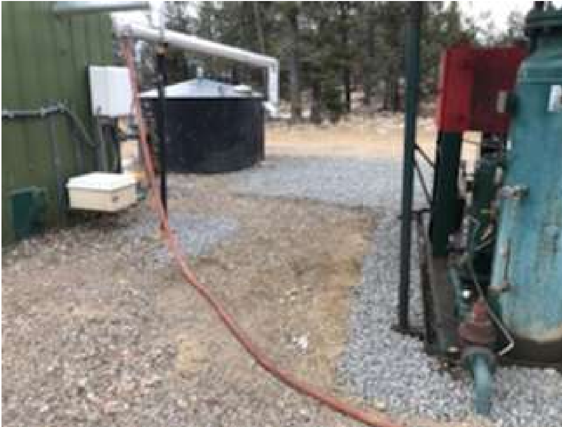
PHOTO 3: THE IMPACTED SOIL NEAR THE LIQUID RING COMPRESSOR WAS REMOVED AND PROPERLY DISPOSED IN ACCORDANCE WITH THE OGRIS OPERATING WASTE MANAGEMENT PLAN.
