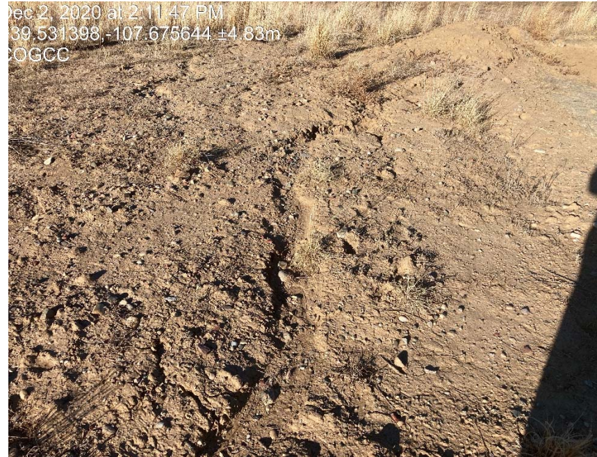
Riling on outside of ditch
