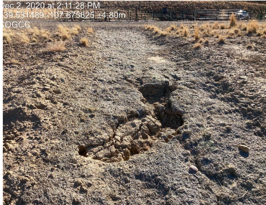
Ditch leading to sediment trap is eroding
