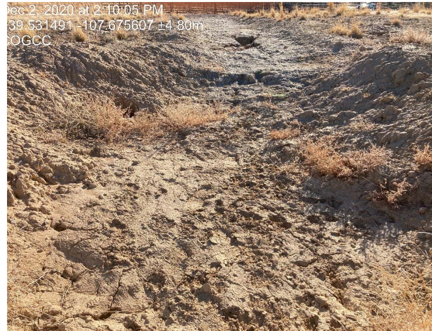
Sediment trap and ditch to pad looking south
