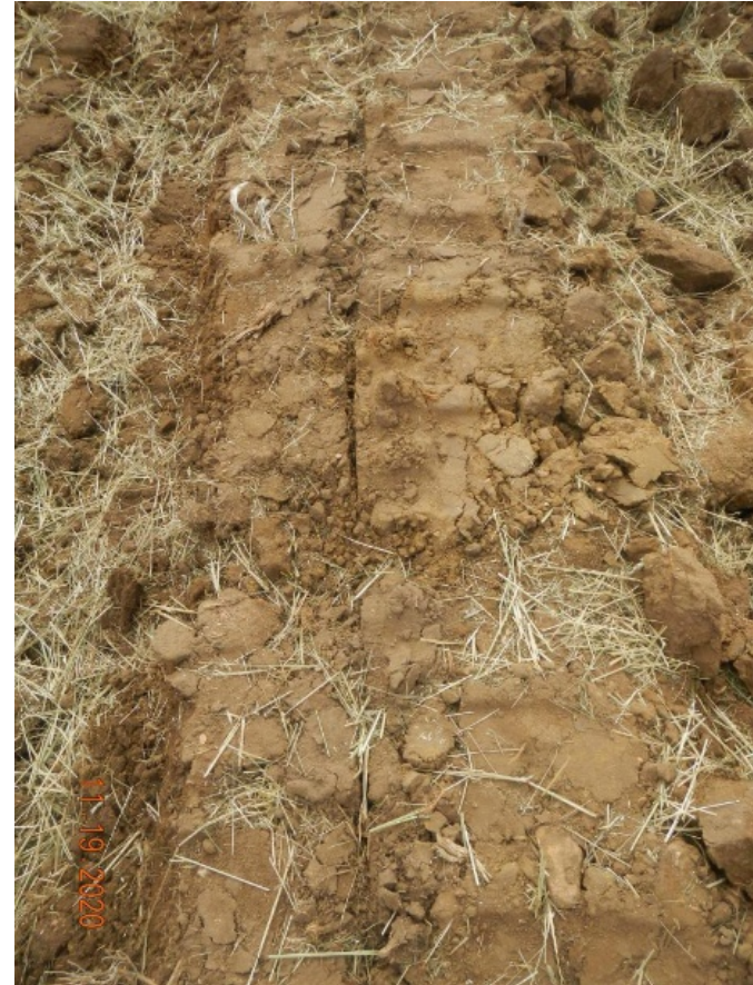
Photo#8: Showing Improper seedbed preparation and stabilization.
