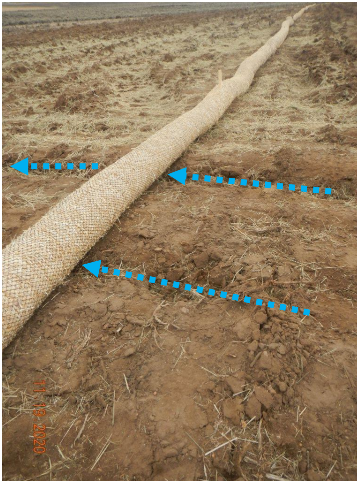
Photo#5: View along West perimeter of Location; improperly positioned and installed wattle. Blue arrows indicate stormwater flow under the wattle.
