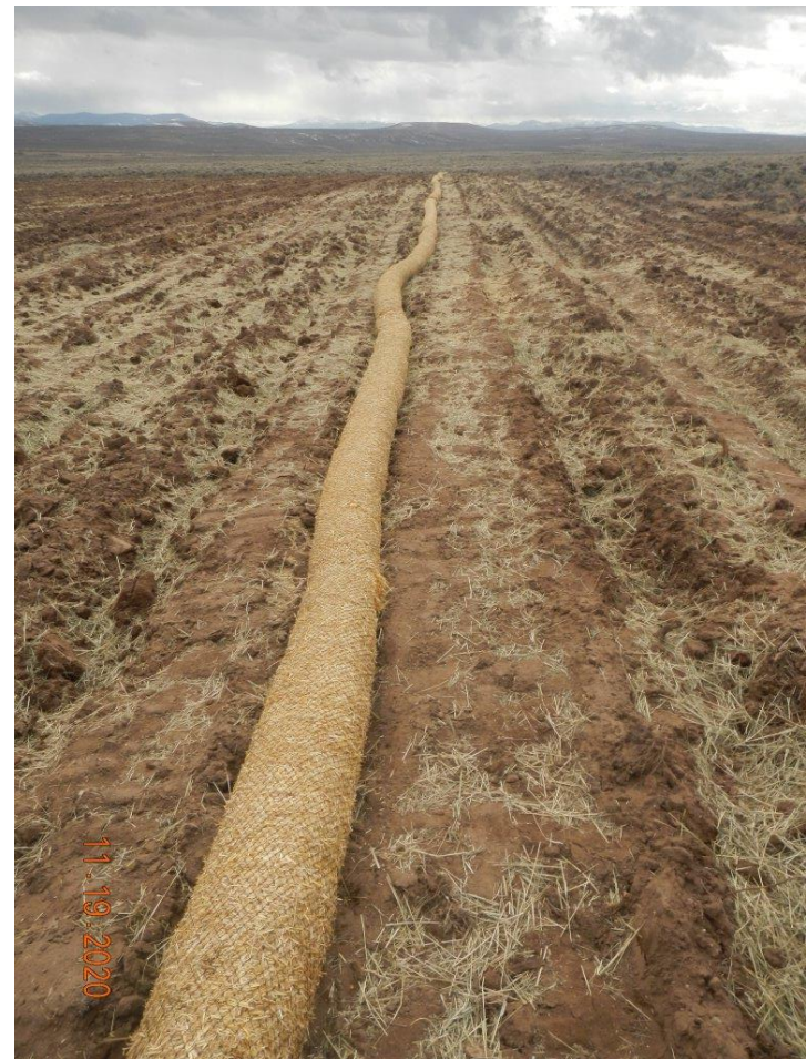
Photo#6: View along West perimeter of Location; improperly positioned and installed wattle.
