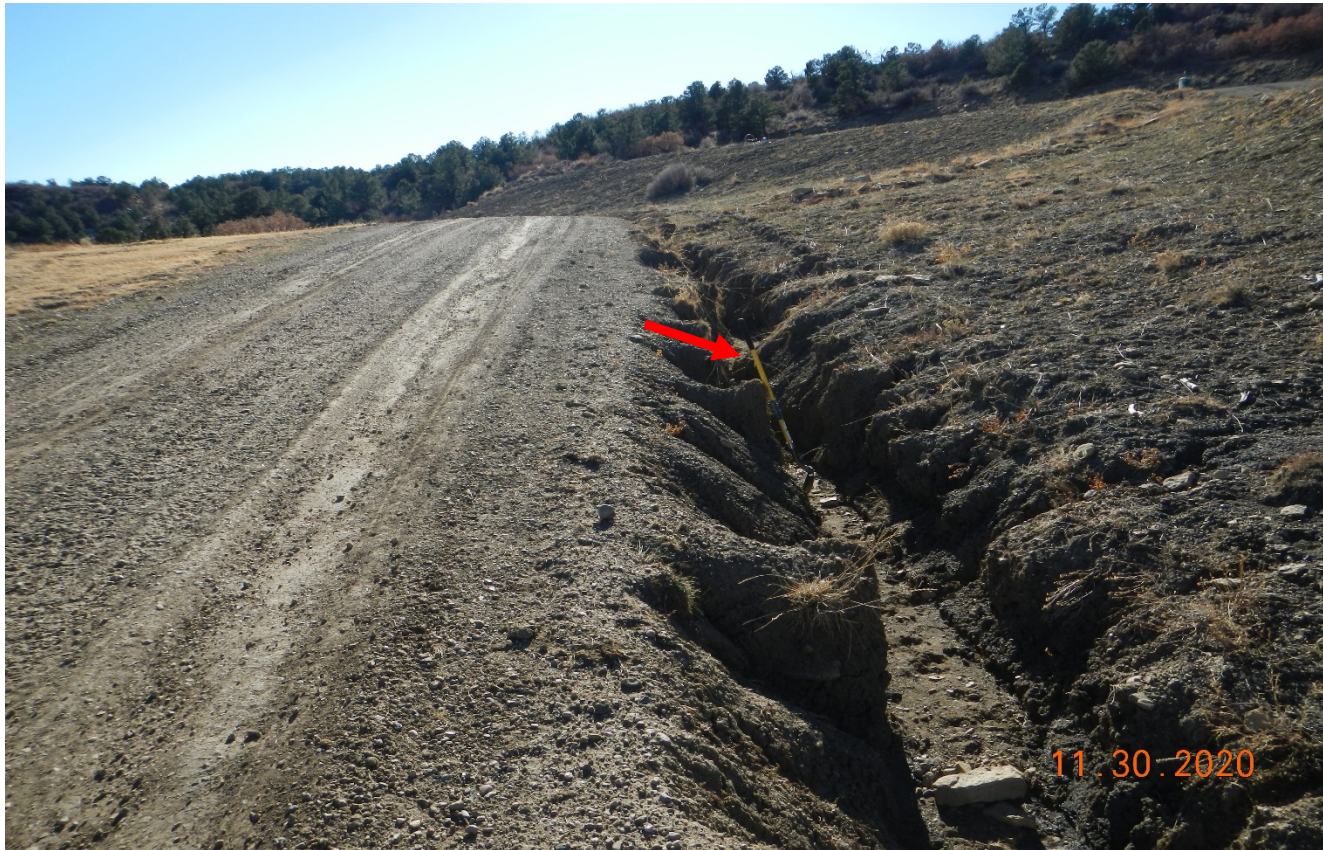
Photo 1. Facing southeast along the main road. The location is at the top of the photo. The red arrow points to 4.5 ft. shovel placed in erosion channel next to the road. Stormwater directed from the location has caused erosion in this area.
