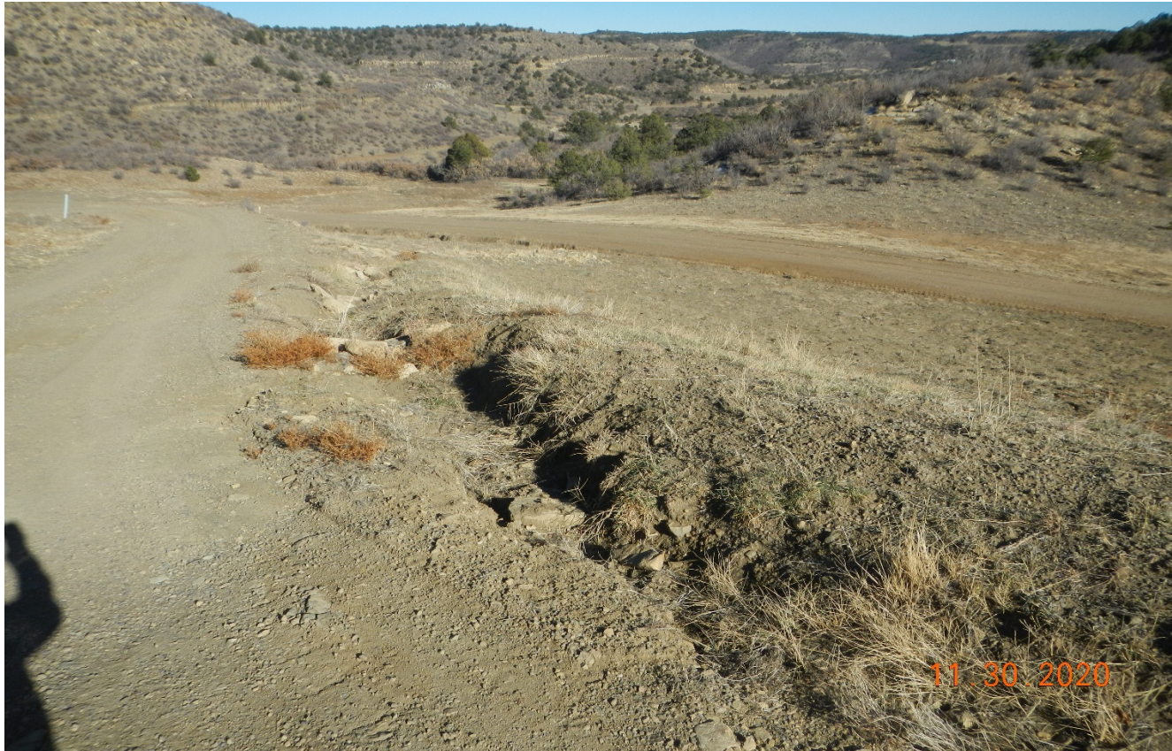
Photo 3. Facing northeast at the access road. Stormwater directed from the location is causing erosion shown in photo 1
