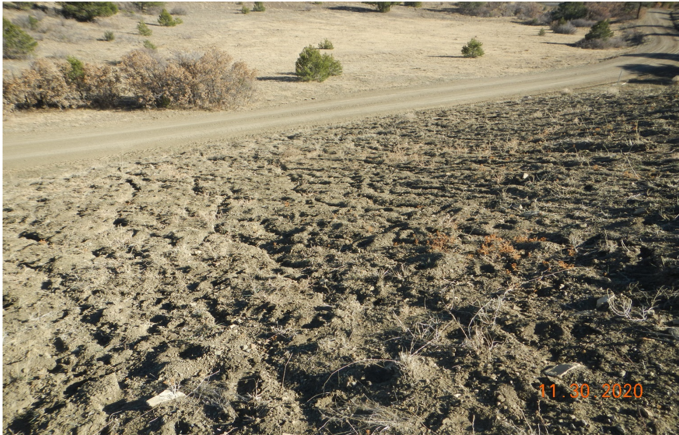
Photo 4. There is erosion rilling occurring along the fill slope of the location.
