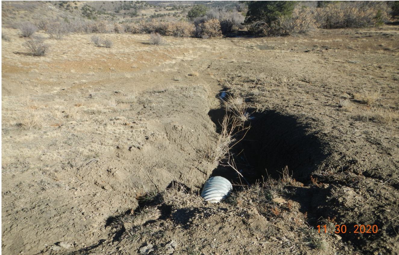
Photo 2. There is erosion occurring at the culvert outlet on the main road near the location.
