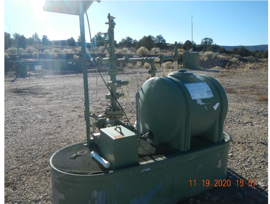
Chemical injection system on secondary containment.
