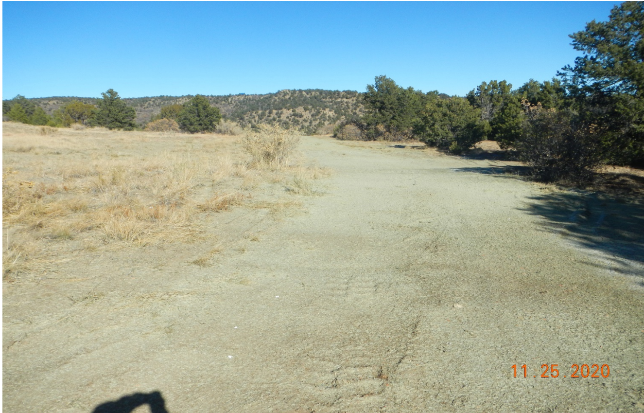
Photo 1. Facing north at beginning of the access road. The bare areas along the road have been seeded and hydromulched.
