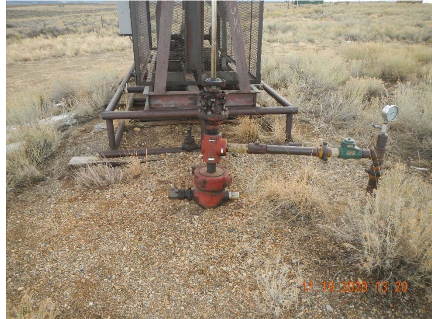
Photo 2. No bradenhead access apparent.
