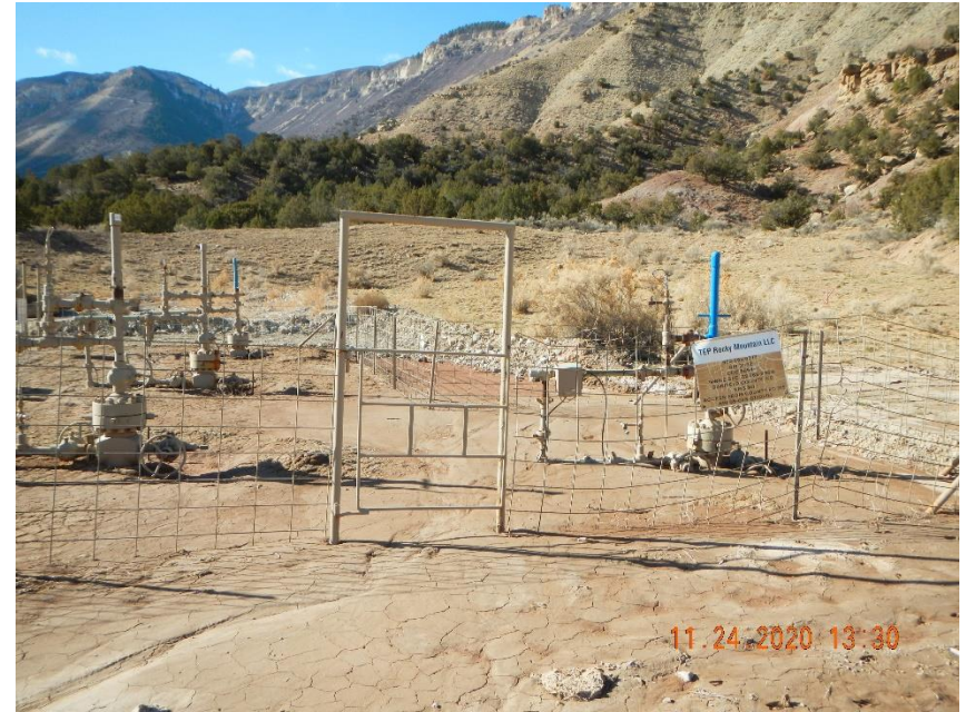
Sediment built up around wells.
