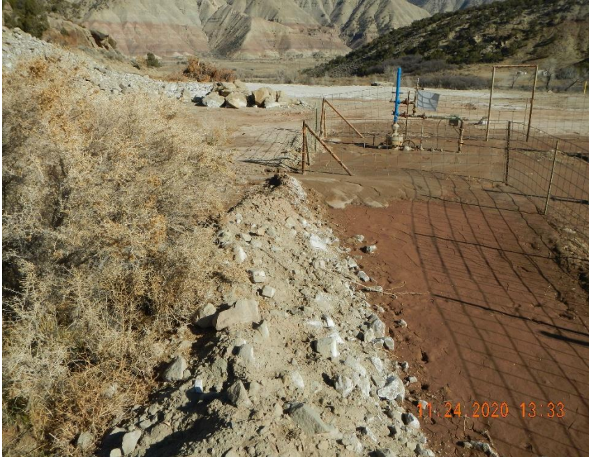
Storm water and sediment flowing to well heads.
