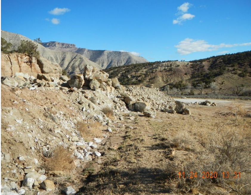
Diversion ditch is blocked off by rock mining.
