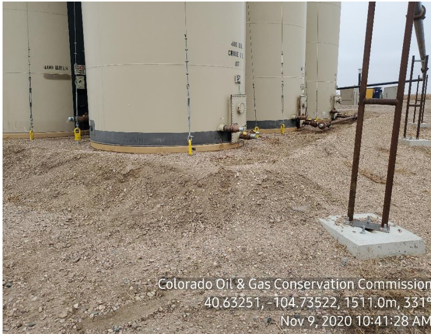
Photo 9: Inadequate berm surrounding tank battery
