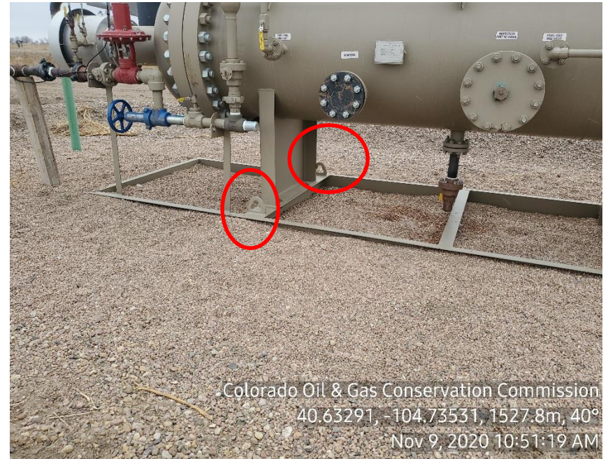
Photo 10: Separator not anchored
