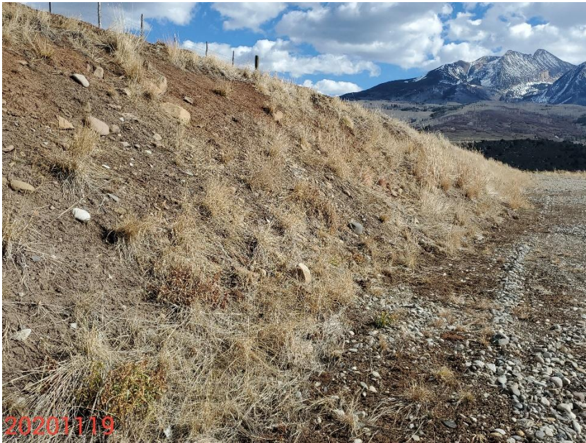
Photo 9: Photo taken from the cut slopes on the northeast end of the Location, facing east. Photo shows BMPs to protect and stabilize the slopes remaining missing or insufficient.
