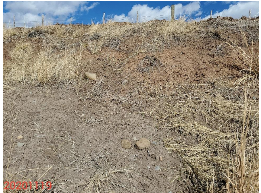
Photo 10: Photo taken from the cut slopes on the northeast end of the Location, facing northeast. Photo shows BMPs to protect and stabilize the slopes remaining missing or insufficient.
