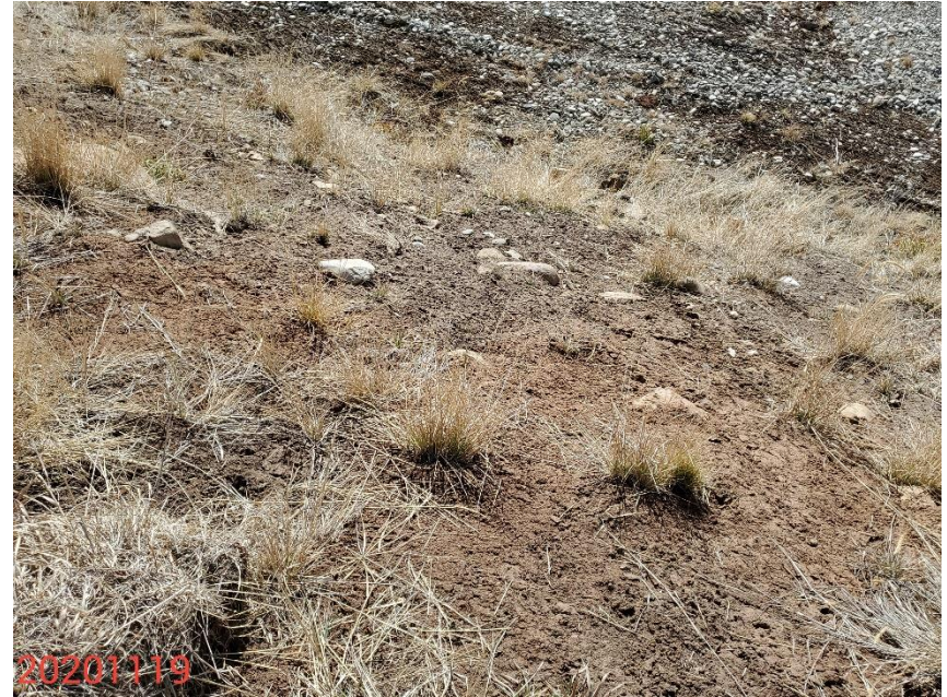
Photo 6: Photo taken from the cut slopes on the northeast end of the Location, facing southwest. Photo shows BMPs to protect and stabilize the slopes remaining missing or insufficient.
