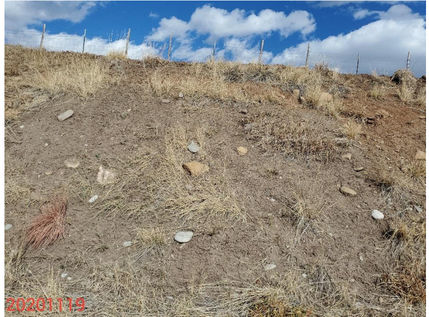
Photo 8: Photo taken from the cut slopes on the northeast end of the Location, facing northeast. Photo shows BMPs to protect and stabilize the slopes remaining missing or insufficient.
