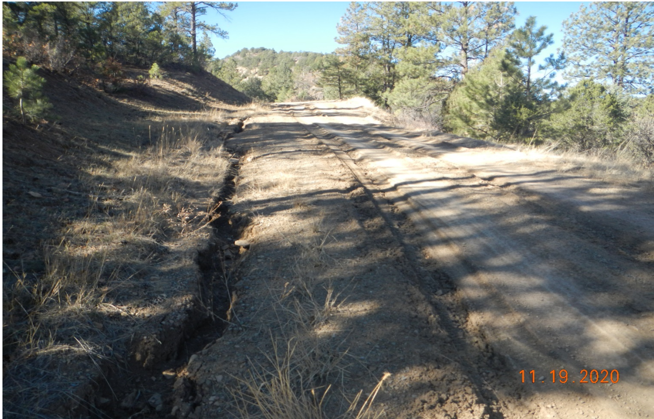
Photo 3. Storm water erosion is occurring down the side of the road. BMP's need to be installed to prevent erosion.
