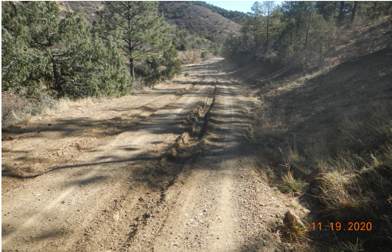
Photo 2. Facing back down the access road shows vehicle rutting. This issue has previously been documented and needs to be repaired and prevented.
