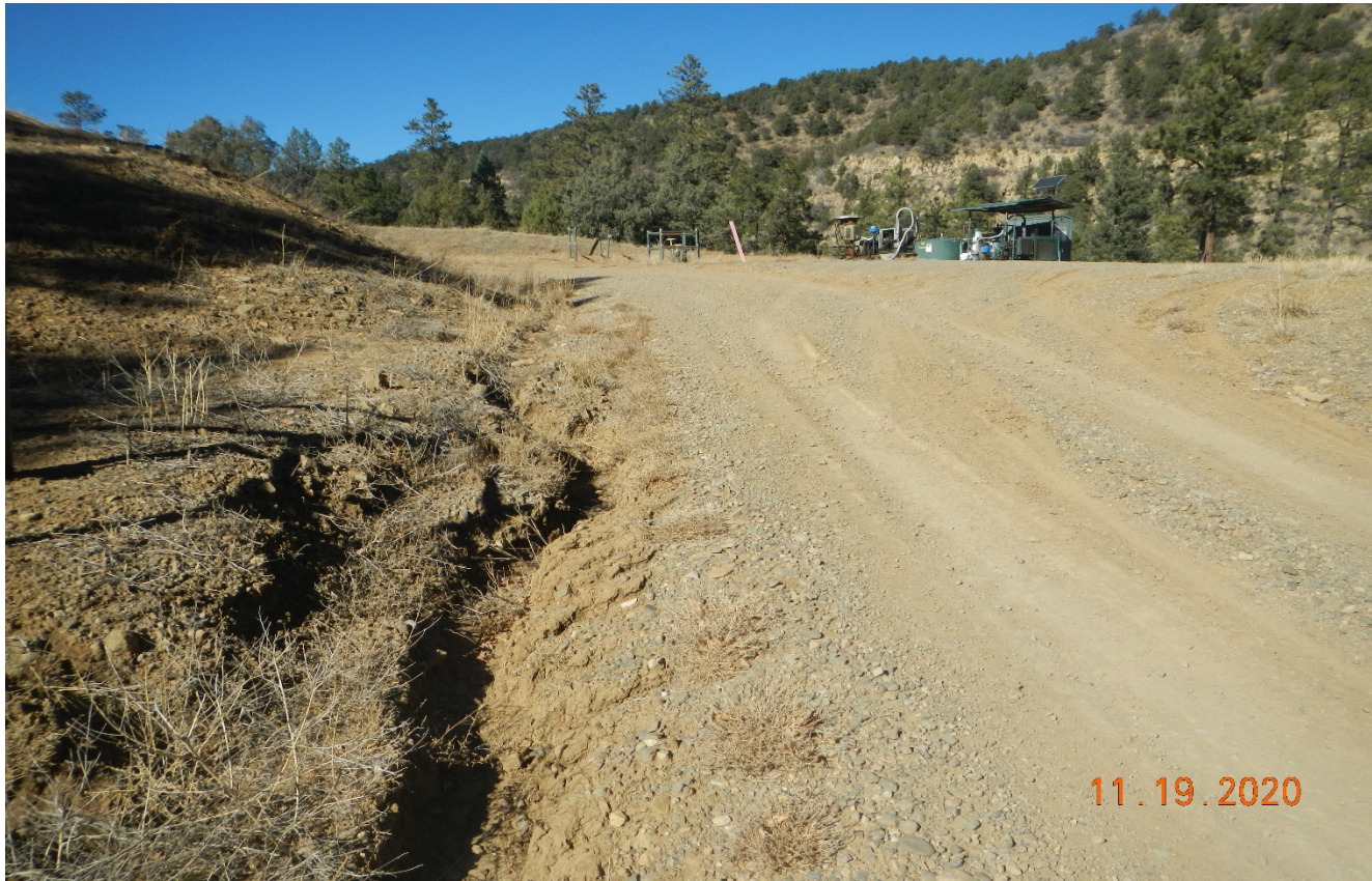
Photo 4. Facing toward the location. Storm water erosion is occurring down the side of the road. BMP's need to be installed to prevent erosion.
