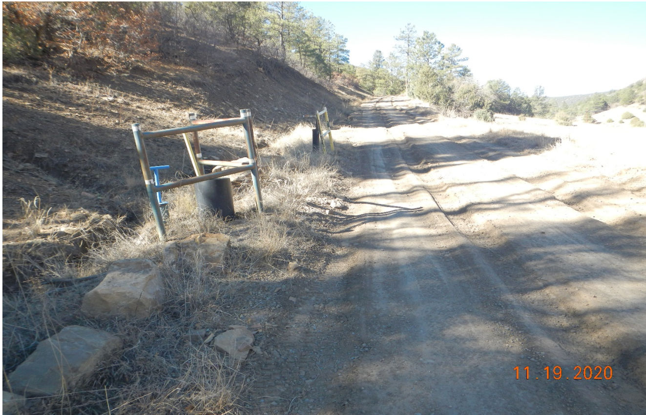
Photo 1. There is vehicle rutting at the beginning of the access road from the main road in Bingham Canyon. This section of road is directing stormwater down the road to the main road. BMP's such as gravel and water bars are needed to prevent rutting and road degradation.
