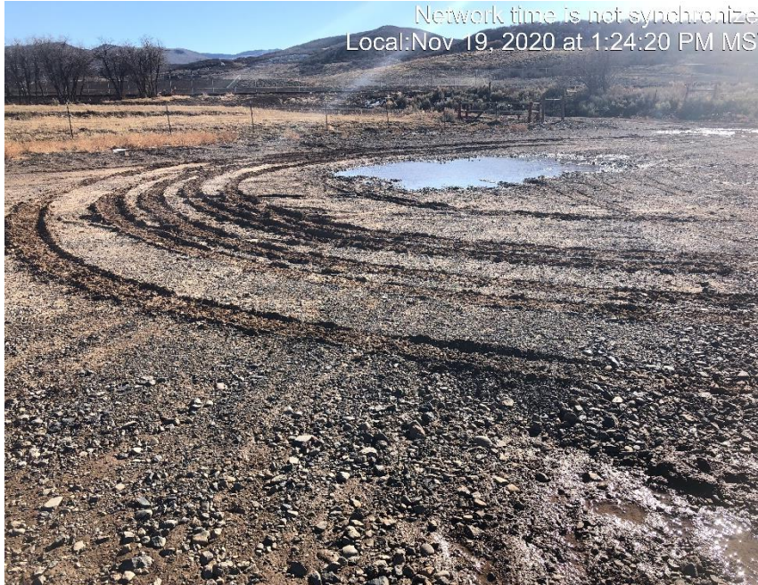
Photo #2293 Rutting occurring due to lack of stabilization.
