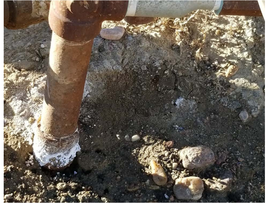
Salt crystals around piping.
