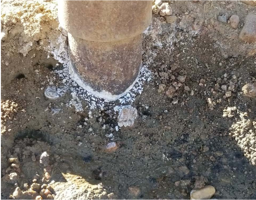
Salt crystals around surface casing.
