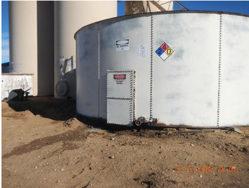
Photo 5. Leak occurring at bolted tank. Dark soil is wet from leaking fluid.
