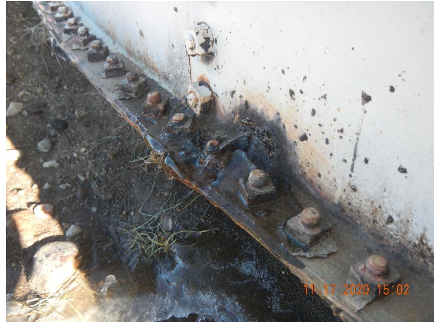
Photo 6. Close up of ongoing leak from photo 5.
