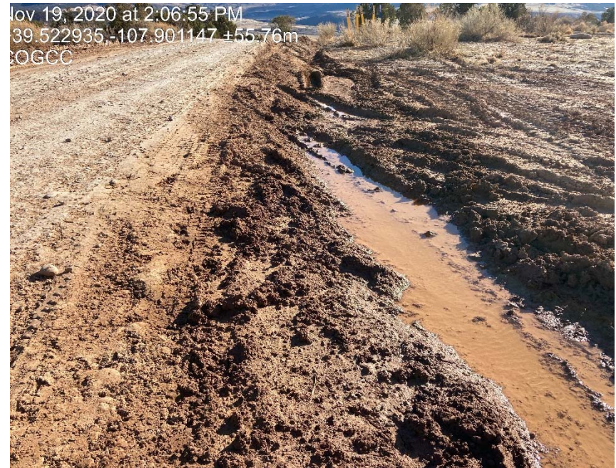
Lack of stabilization leading to tracking
