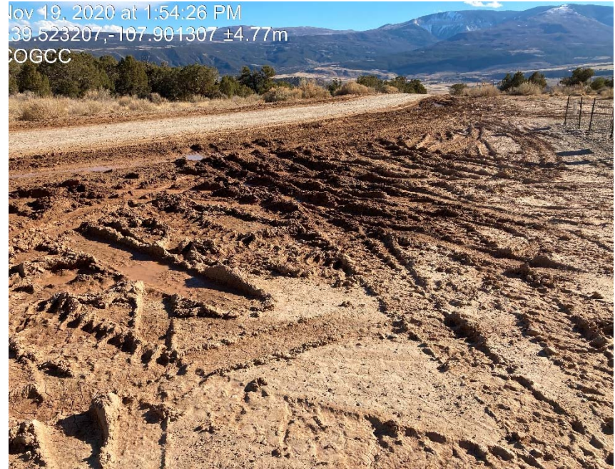
Lack of stabilization leading to tracking
