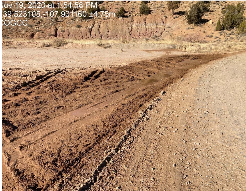
Lack of stabilization leading to tracking
