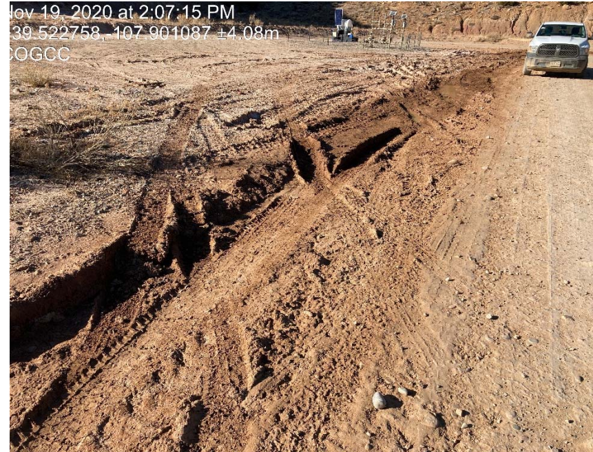
Lack of stabilization leading to tracking
