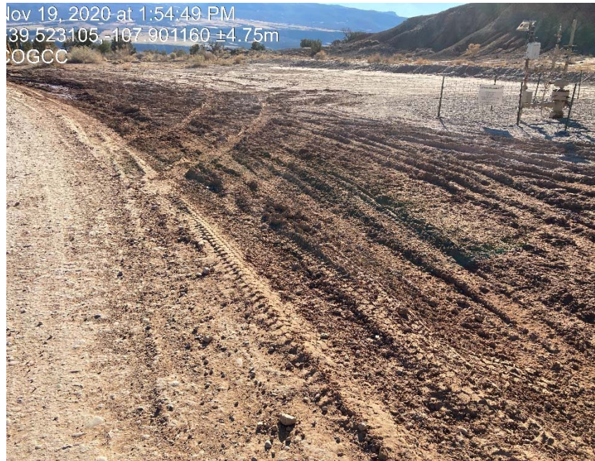
Lack of stabilization leading to tracking
