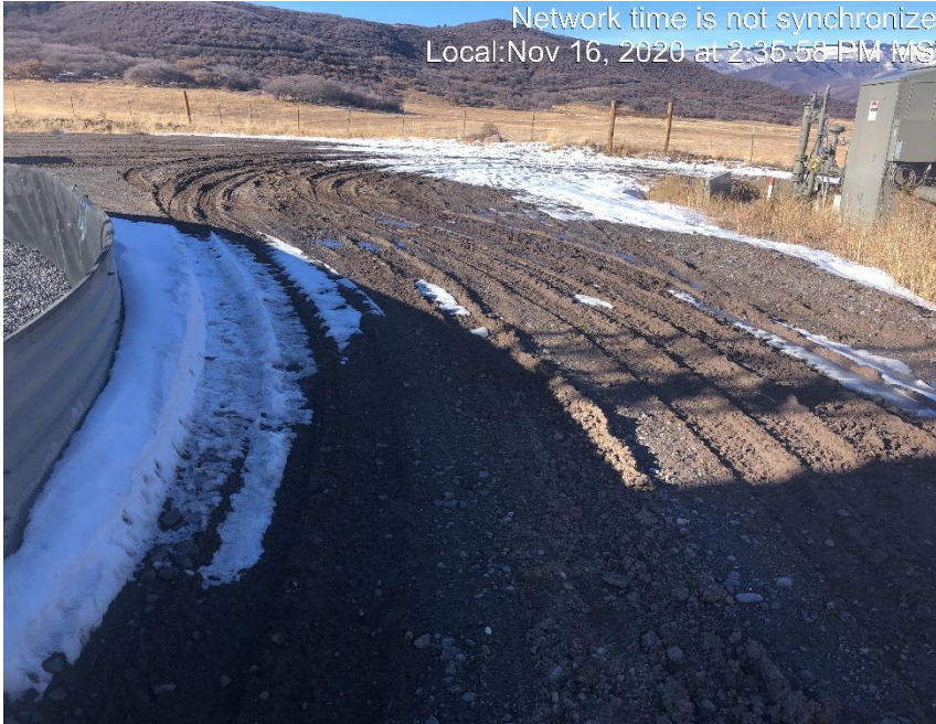
Photo #2259 Sediment migrating off of location and on to access road due to tracking.
