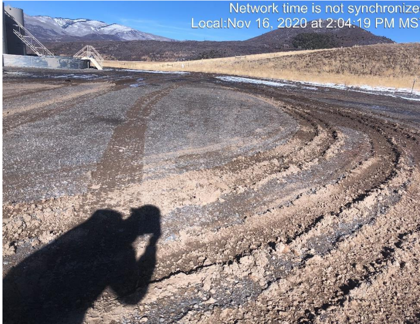
Photo #2250 Sediment migrating off of location and on to access road due to tracking.
