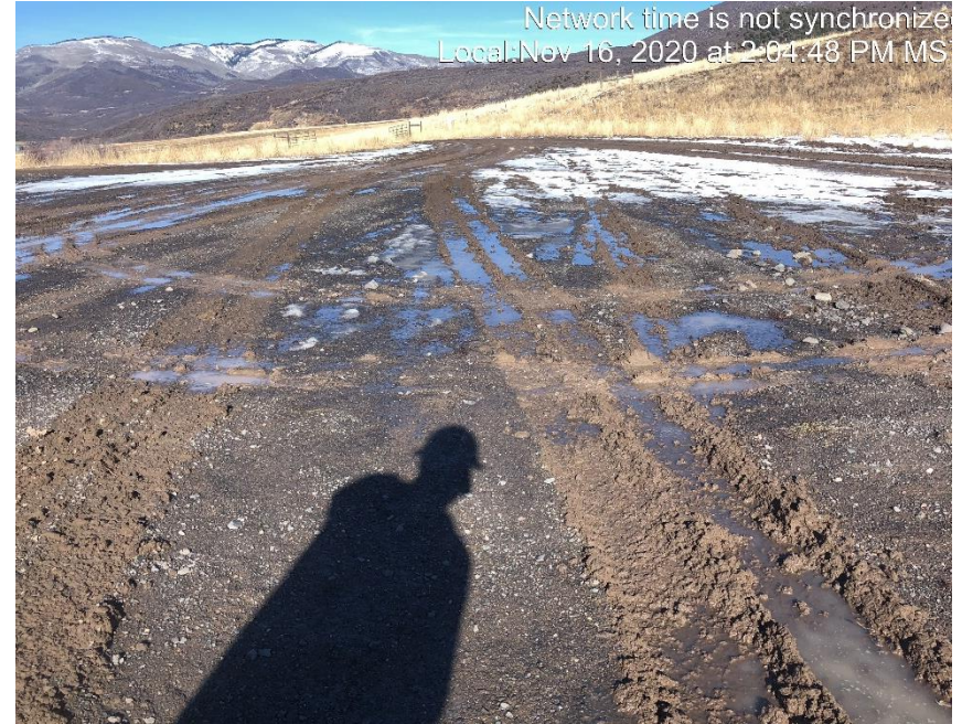
Photo #2251 Sediment migrating off of location and on to access road due to tracking.
