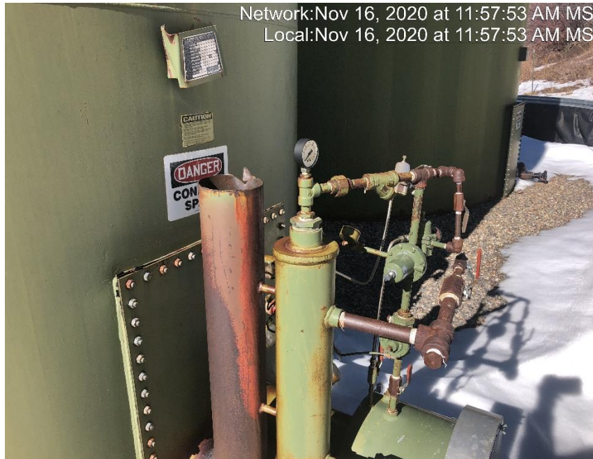
Photo #2239 Tank burner assembly missing bird protector.
