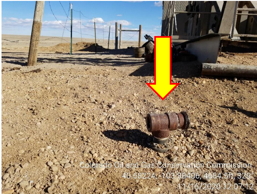
Photo 3 – Unmarked Riser at Wellhead
