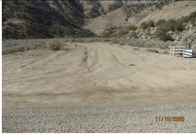
Erosion Channels and Vehicle Ruts on the Oxy Fed 797-08-51D Access Road
