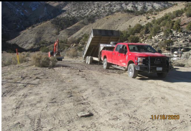
Shale Installed on the Oxy Fed 797-08-51D Access Road
