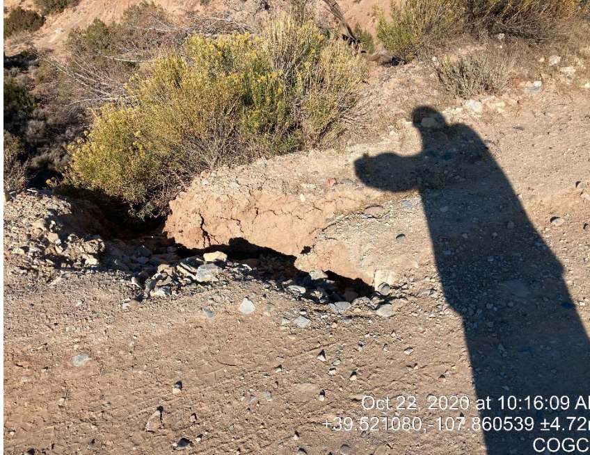
Main road to access pad erosion. At top of hill just before compressor station.
