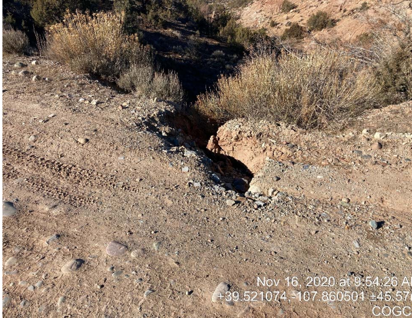
Recent inspection of Main road to access pad erosion. At top of hill just before compressor station.
