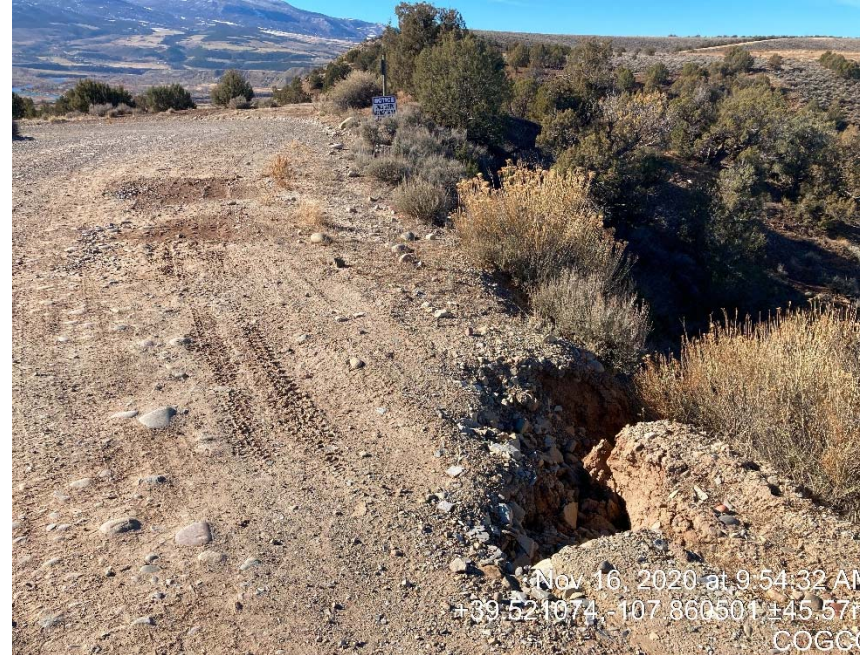
Recent inspection of Main road to access pad erosion. At top of hill just before compressor station.
