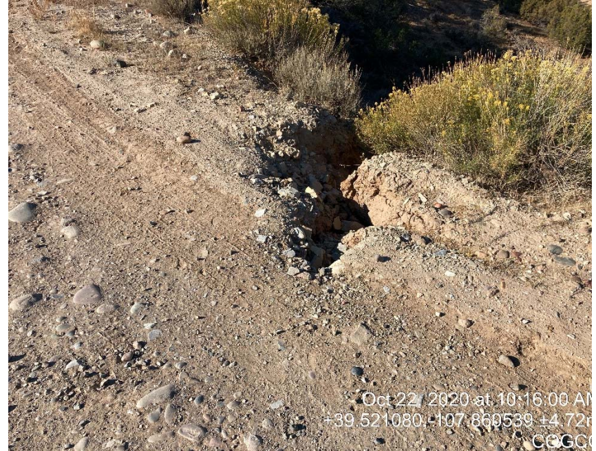
Main road to access pad erosion. At top of hill just before compressor station.
