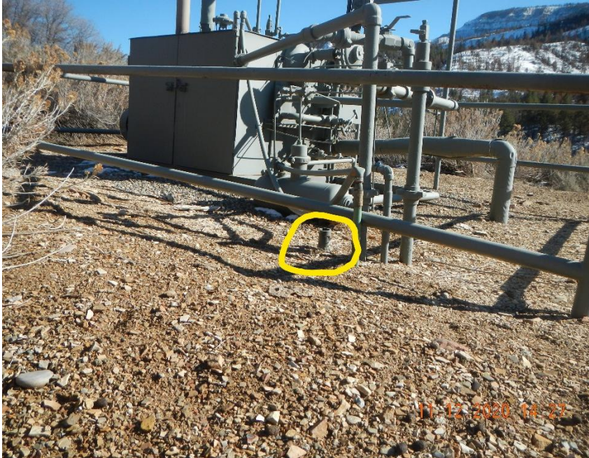
Unused 2" flow line risers at separator.
