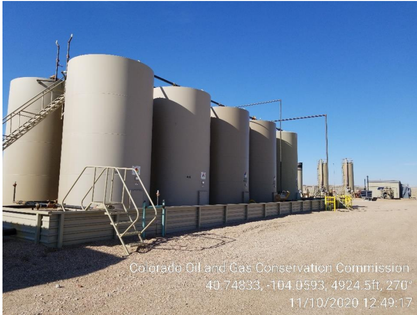
Photo 1 – Tank Battery
