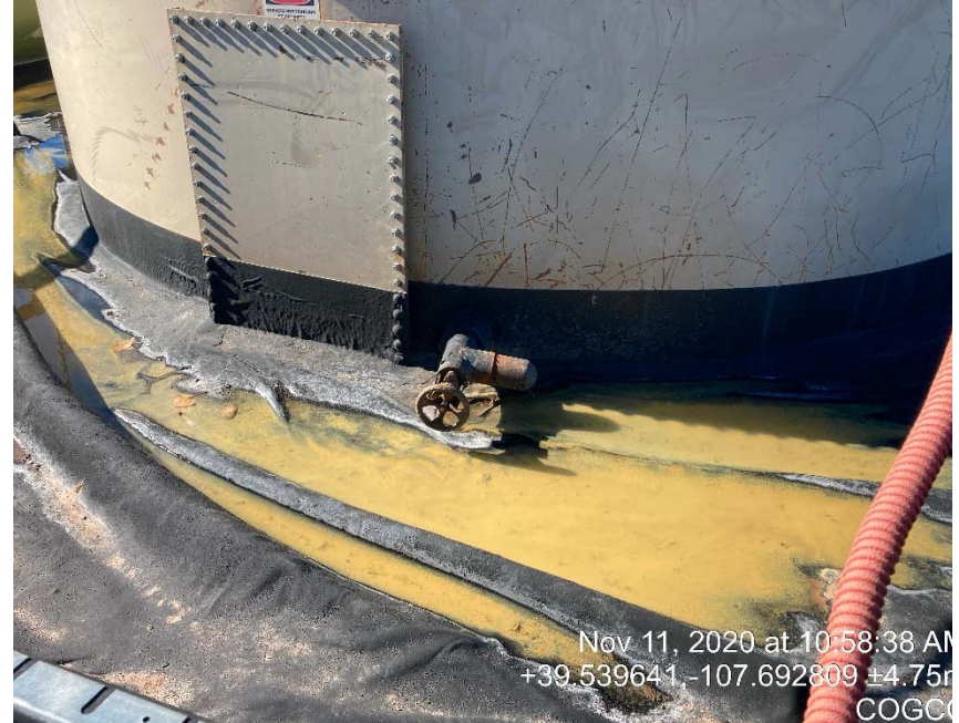
Leaking Valve
