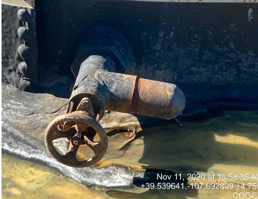
Leaking Valve
