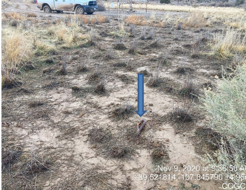
Sediment Migration/choking out vegetation/unmarked dead man
