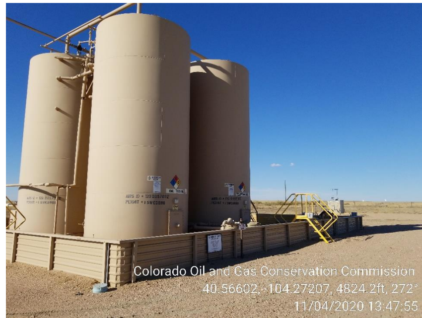
Photo 2 – Tank Battery
