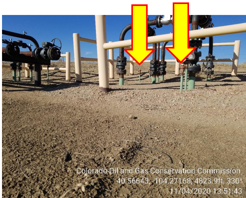
Photo 5 – Unmarked Risers at East end of Rack
