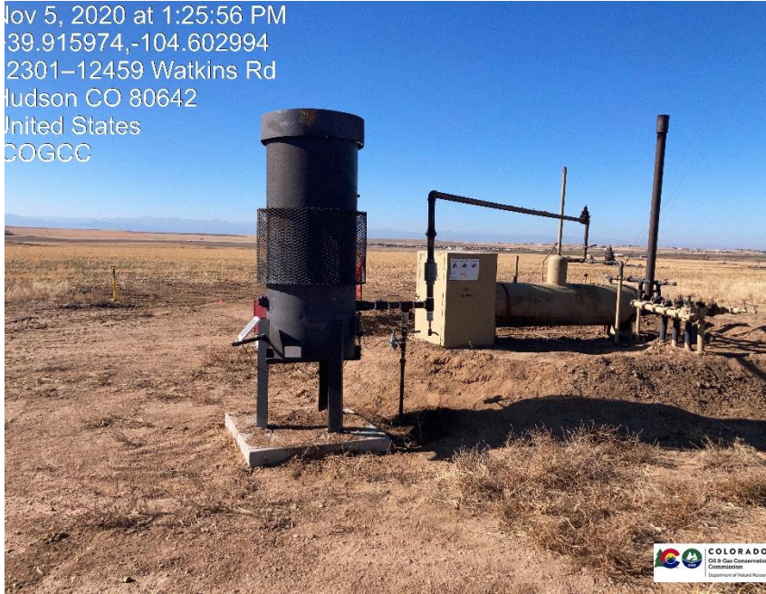
Pic 3 ECD flaring produced gas on location
