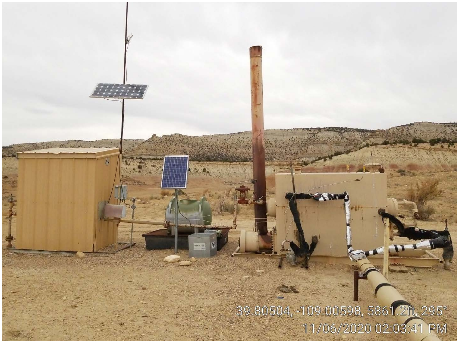
Photo 2. Meter building & separator.
