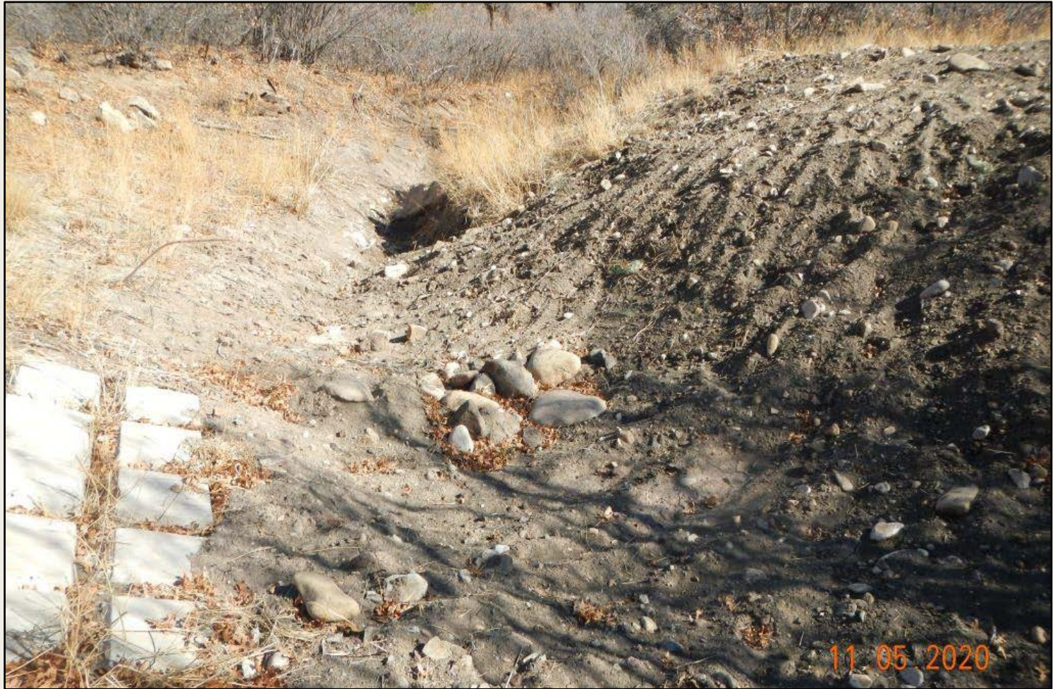
Photo 2. View of work conducted where erosional head-cut was observed during an earlier reclamation inspection. Bare soils are not protected, and will likely rapidly erode.
