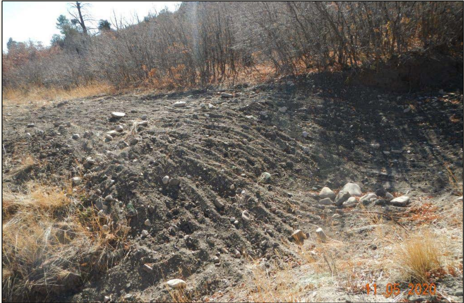
Photo 3. View of disturbed soils at the bank of erosional repair. Seeding is not apparent.
