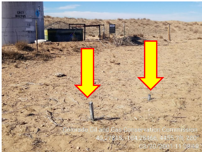
Photo 7 – NW Deadman Anchors NOT Marked
