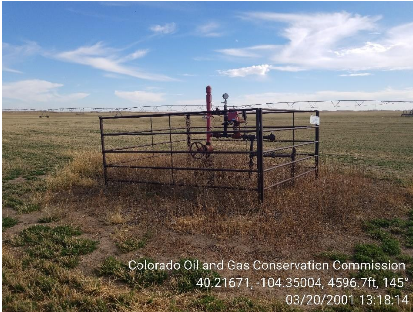
Photo 1 – Wellhead, WEEDS
