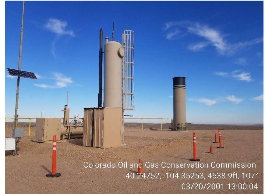
Photo 4 – Heater Treater, Separator, ECD
