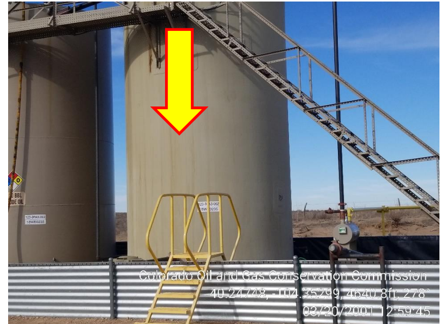
Photo 6 – Produced Water Tank missing – NFPA, Content, and Capacity
