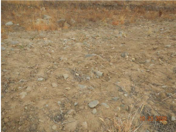
Photo#4: Initiation of erosion on Fill Slope.
