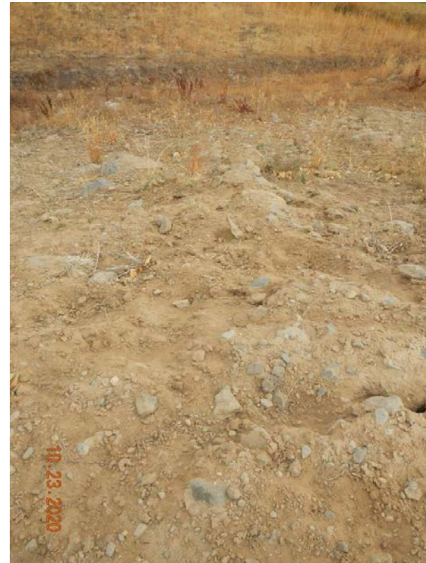
Photo#5: Initiation of erosion on Fill Slope.
