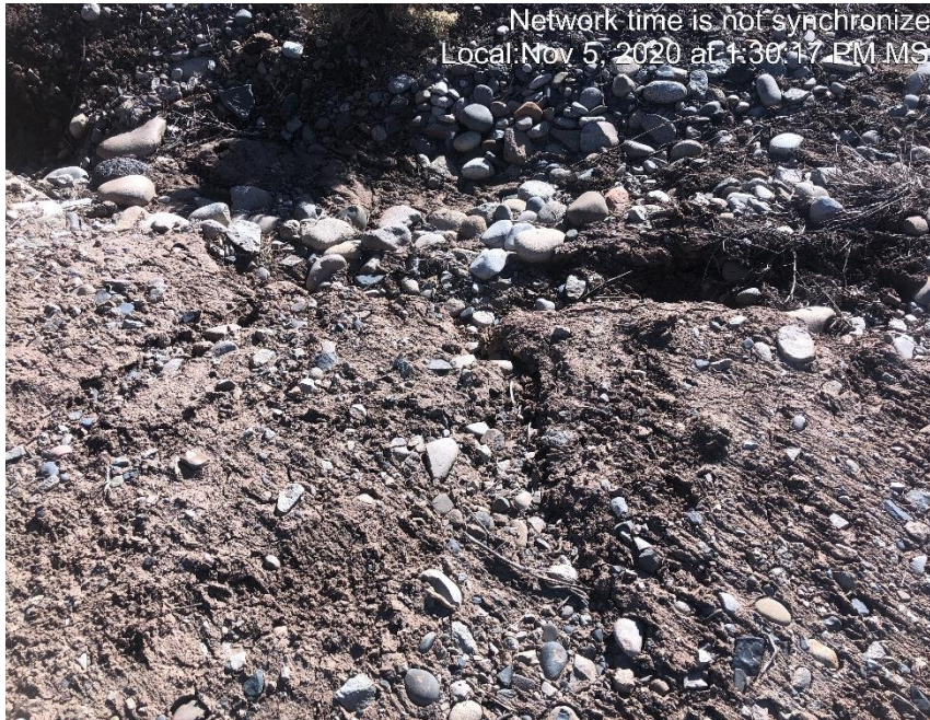
Photo #2207 Rill erosion occurring in ditch at inlet to culvert.
