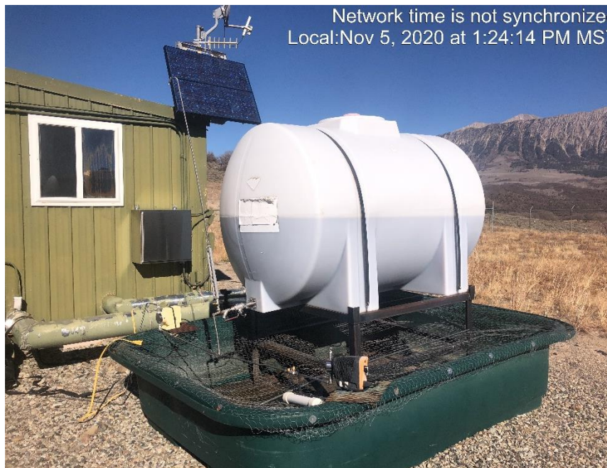
Photo #2200 Chemical tank NFPA label weathered and not legible.
