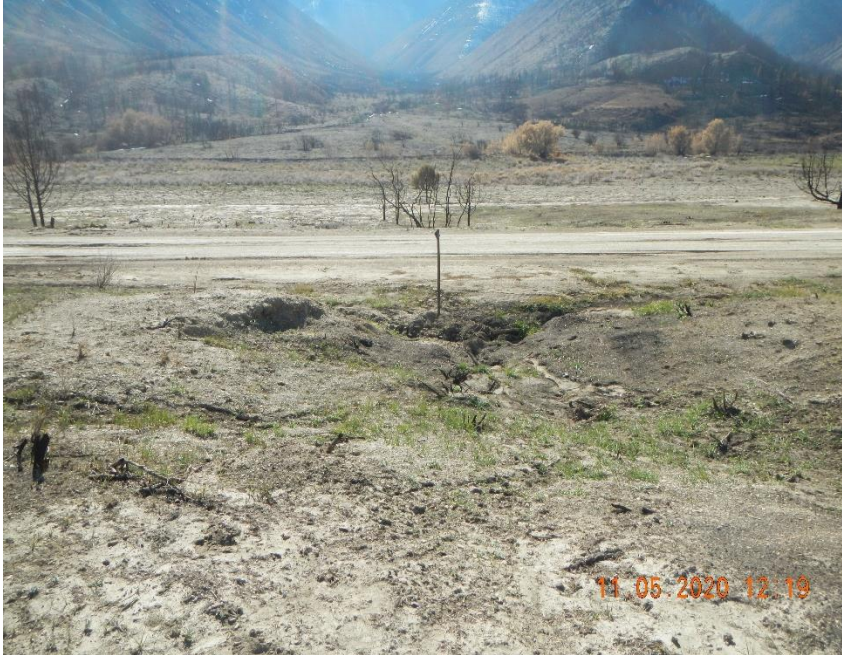
Sediment covering culvert inlet.
