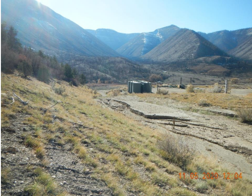
Sediment buildup in diversion ditch.
