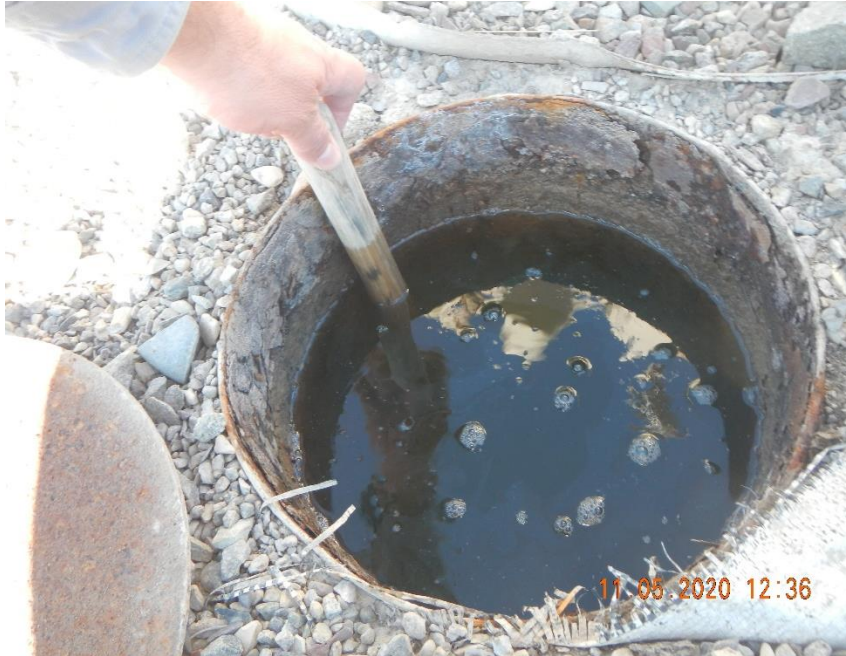
Loose lid on unbackfilled rat hole.
