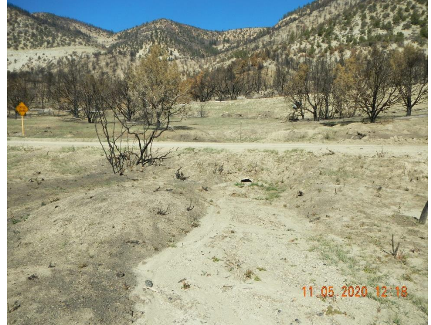
Culvert outlet packed off.
