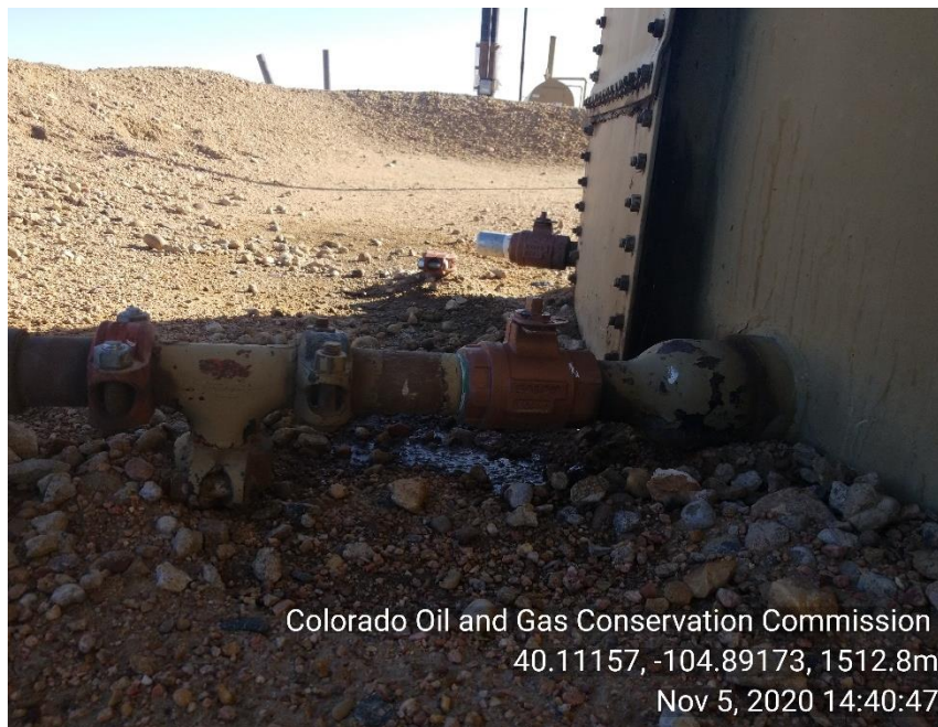
Photo 10 2" line on crude oil tank actively leaking.
