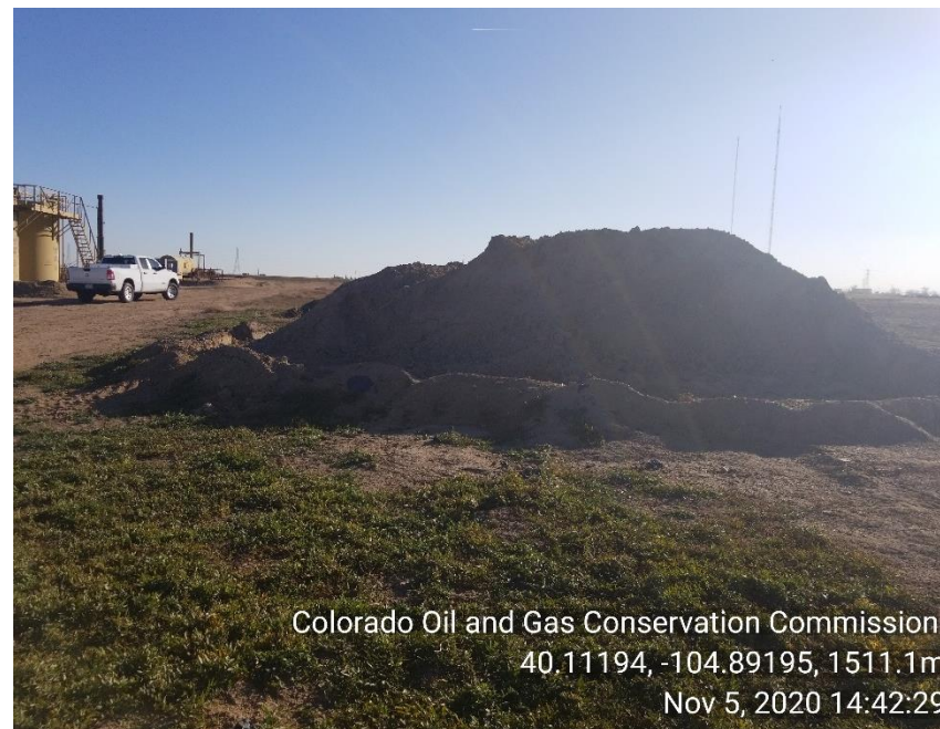
Photo 13 BMP around material from spill remediation not adequate.
