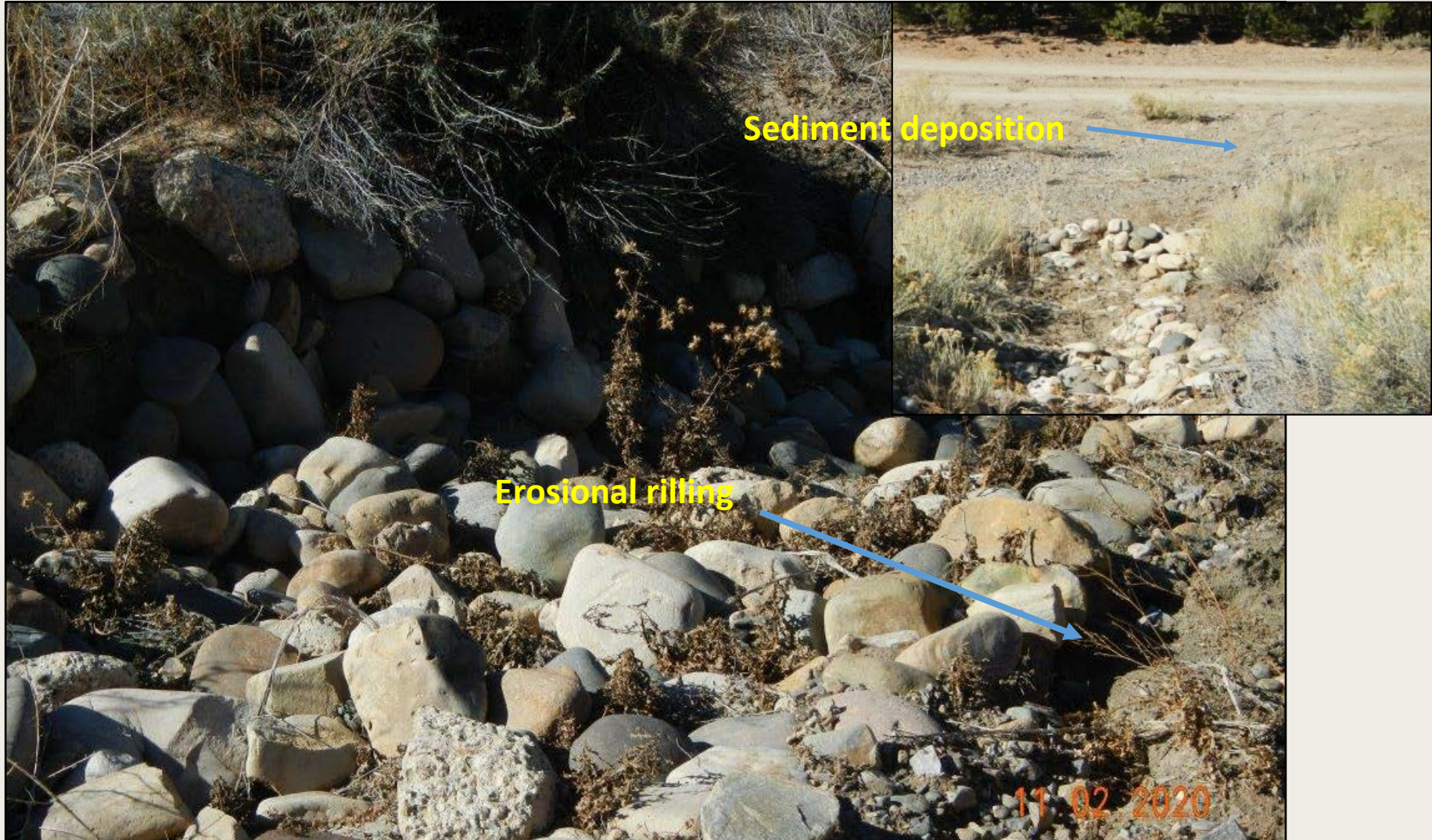
Photo 3. View of cobble run-down in the northern project area. Erosional rilling is occurring around cobbles. Sediment deposition observed at the bottom of the slope (inset). Canada thistles appear to be herbicide treated.
