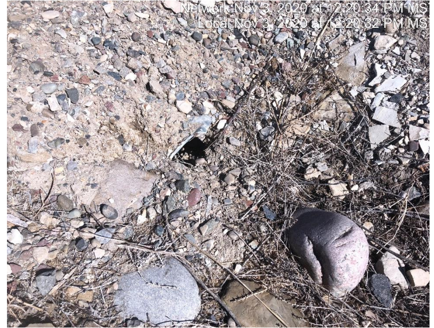
Photo #2176 Culvert inlet and outlet blocked by sediment.
