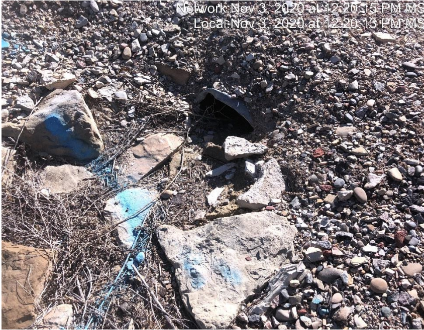
Photo #2175 Culvert inlet and outlet blocked by sediment.
