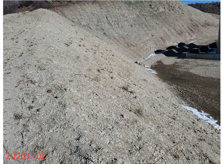
Photo 2: Photo taken from the west end of the Location, facing northeast. Photo shows BMPs remain missing or insufficient to stabilize the cut slopes on the western ends of the Location.
