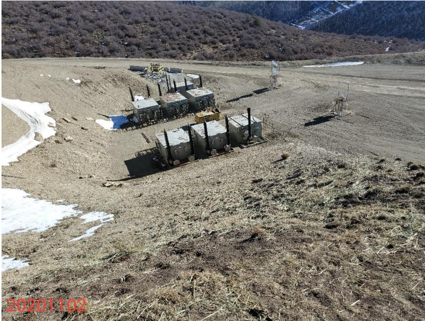
Photo 7: Photo taken from the north end of the Location, facing east. Photo shows BMPs remain missing or insufficient to stabilize the cut slopes on the north ends of the Location.
