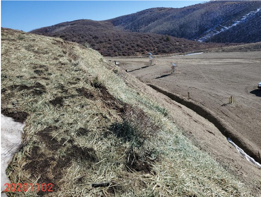
Photo 5: Photo taken from the north end of the Location, facing northeast. Photo shows remnants of mulch that was applied to the northern slopes behind the tank battery. Photo shows BMP is insufficient to stabilize the slopes on the north end of the Location.
