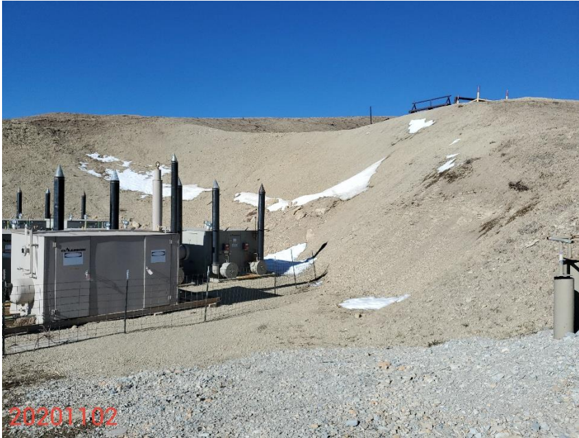
Photo 9: Photo taken from the northeast end of the Location, facing west. Photo shows BMPs remain missing or insufficient to stabilize the cut slopes on the north ends of the Location.
