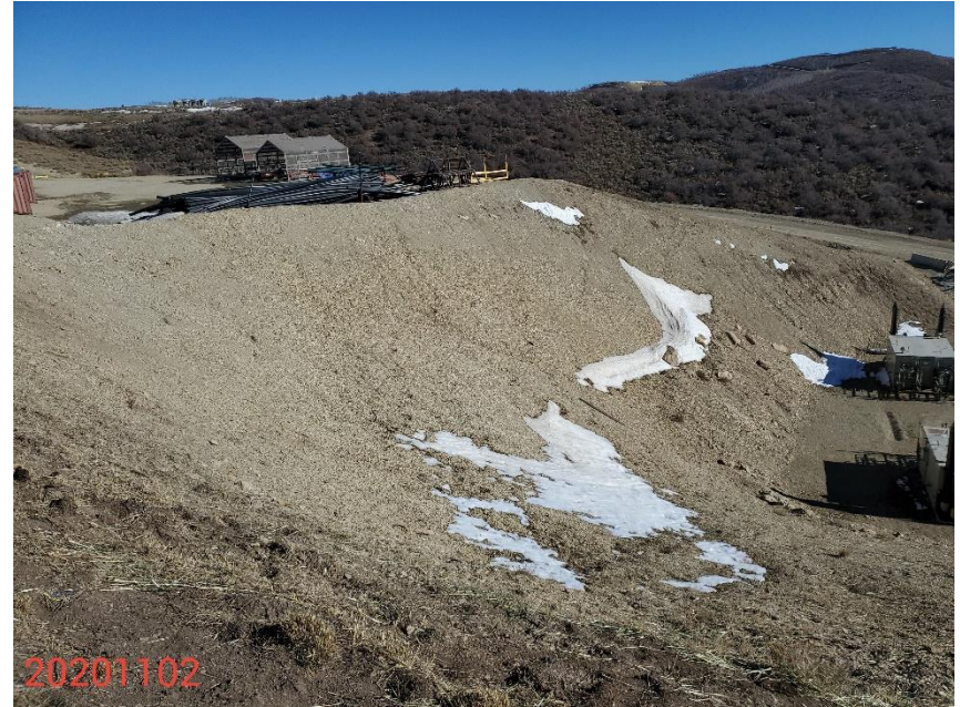
Photo 6: Photo taken from the north end of the Location, facing northeast. Photo shows BMPs remain missing or insufficient to stabilize the cut slopes on the north ends of the Location.
