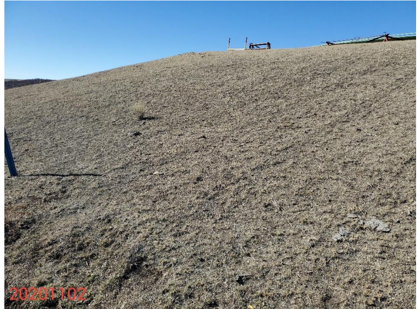
Photo 10: Photo taken from the access road, facing west. Photo shows interim slopes below the "storage area". Photo shows Operator has installed erosion netting to help stabilize the slopes east and west of the "storage area". BMP appears to be in proper functioning condition.
