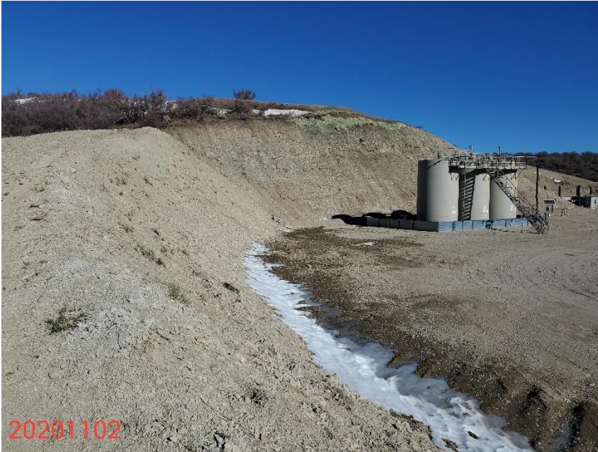
Photo 1: Photo taken from the west end of the Location, facing northeast. Photos show BMPs remain missing or insufficient to stabilize the cut slopes on the northern and western ends of the Location.
