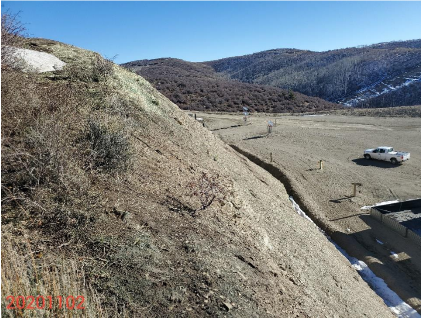
Photo 3: Photo taken from the northwest corner of the Location, facing northeast. Photo shows BMPs remain missing or insufficient to stabilize the slopes on the north end of the Location.
