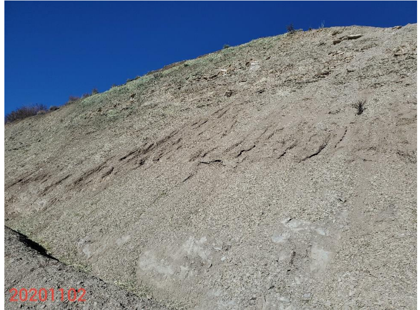
Photo 8: Photo taken from the north end of the Location, facing northwest. Photo shows BMPs remain missing or insufficient to stabilize the cut slopes on the north ends of the Location.
