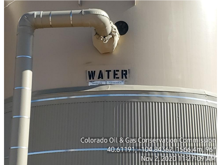
Photo 4: No Capacity or NFPA placard
