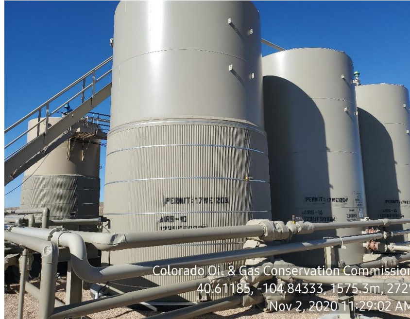
Photo 7: No labeling on tank
