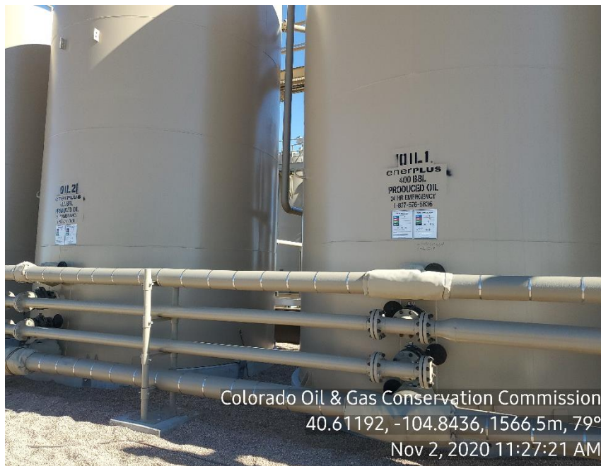
Photo 5: No NFPA placarding on crude oil tanks
