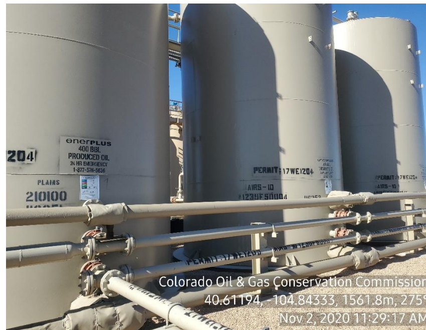
Photo 6: No NFPA placarding on crude oil tanks
