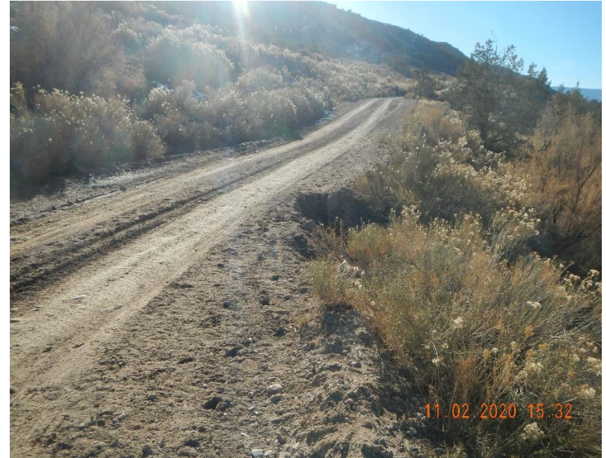
Shoulder of road washing away. GPS Coordinates 39.47161 107.97009
