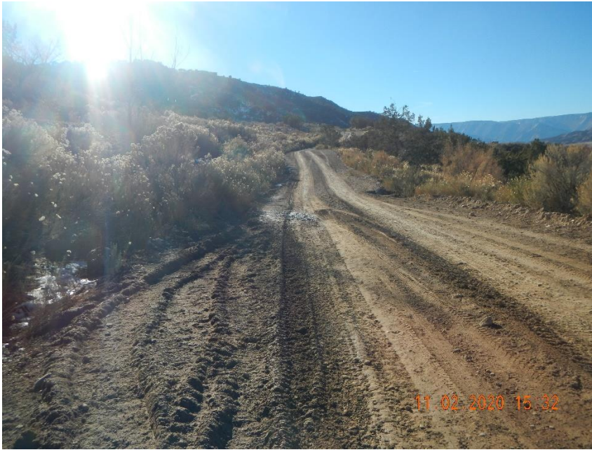
Shoulder of road washing away. GPS Coordinates 39.47161 107.97009
