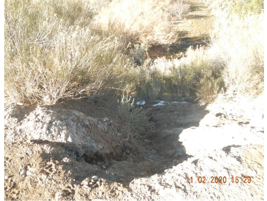
Shoulder of road washing away. GPS Coordinates 39.47161 107.97009
