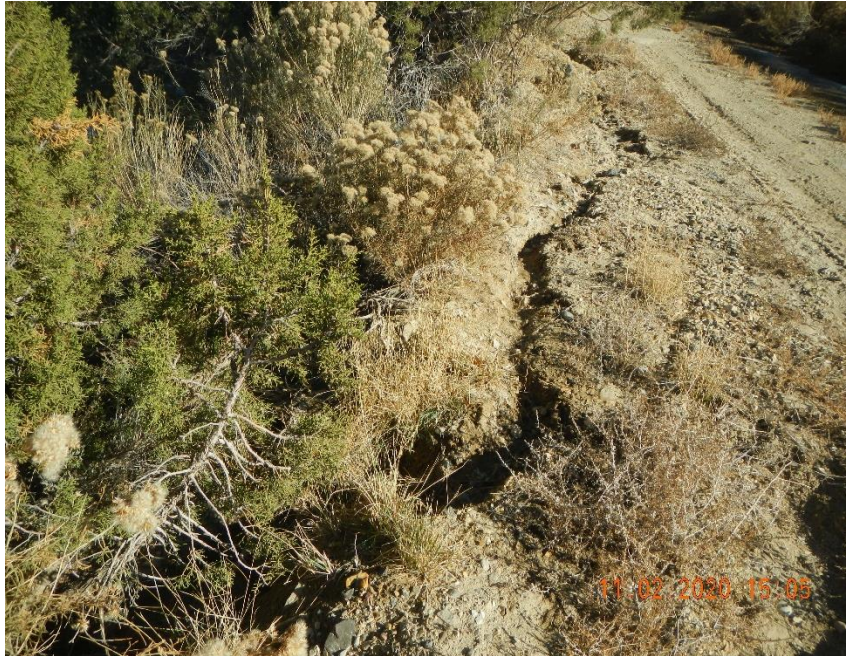
Washing going over shoulder of entrance road near well site. GPS Coordinates 39.47150 107.98080
