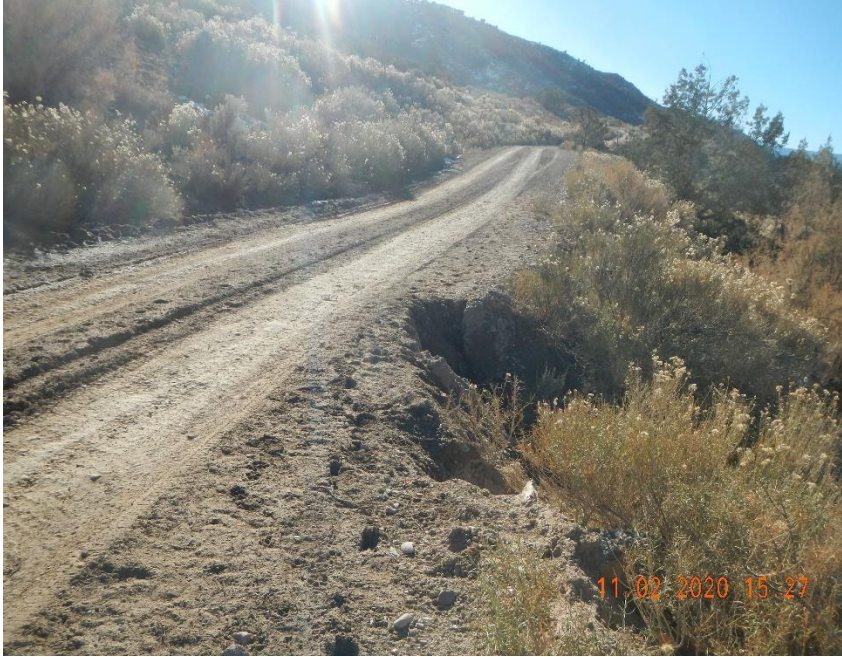
Shoulder of road washing away. GPS Coordinates 39.47161 107.97009
