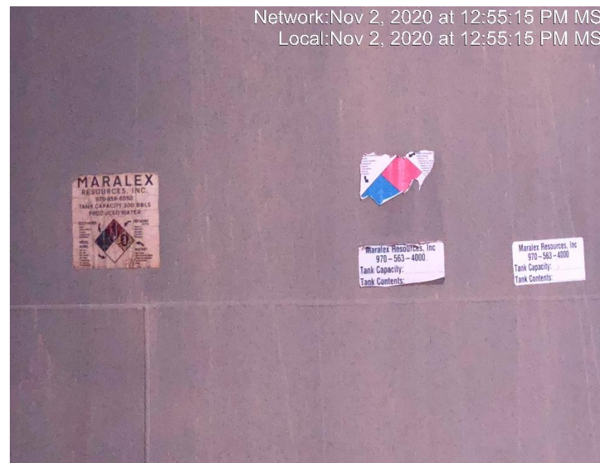
Photo #2164 Tank capacity, contents and NFPA labels weathered and not legible.
