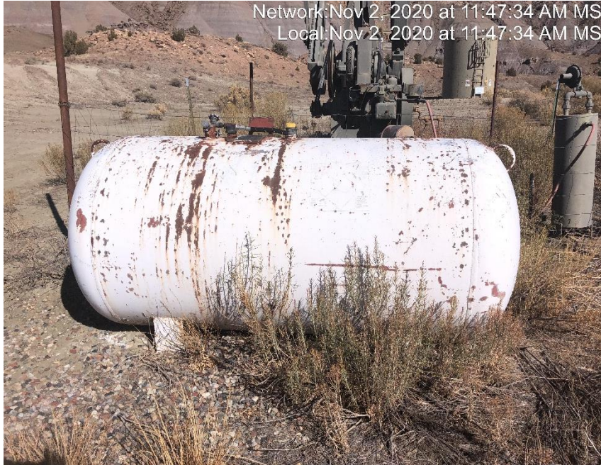
Photo #2156 Tank by wellhead is not properly labeled.
