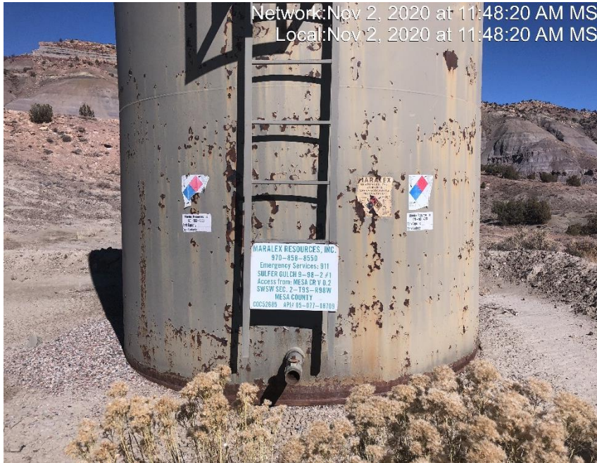
Photo #2157 Tank label and placards are weathered and not legible.
