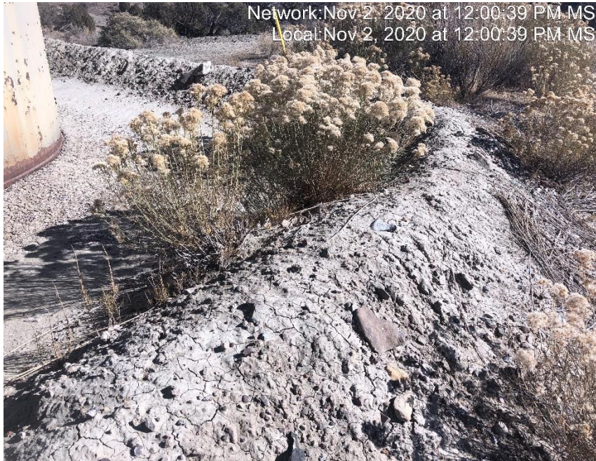
Photo #2159 Vegetation growing on tank containment berm.
