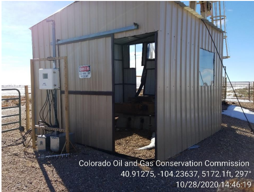
Photo 3 – Gas Engine has been removed
