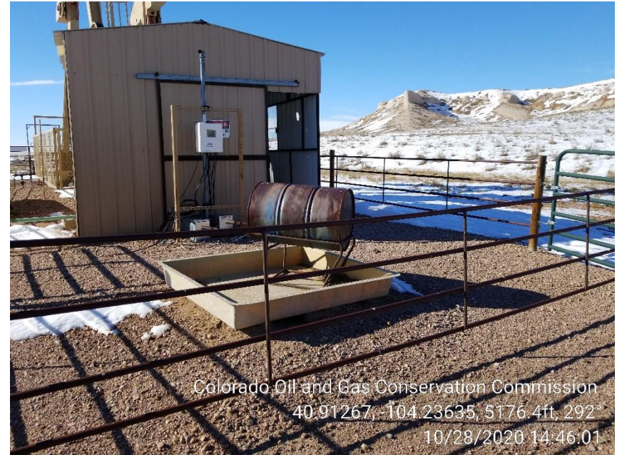
Photo 2 – Unused Chemical Tank and Containment
