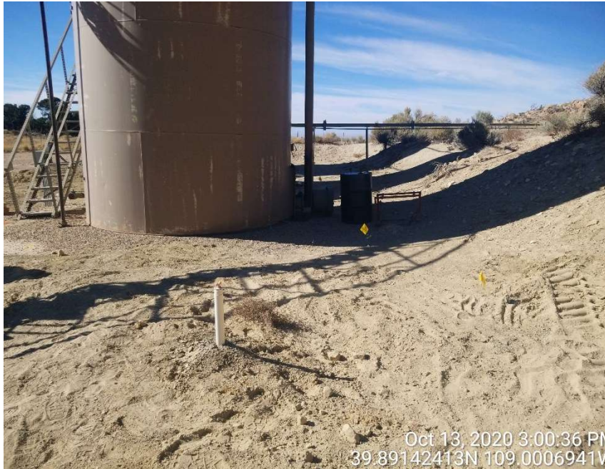
Monitoring well within the tank battery secondary containment structure.
