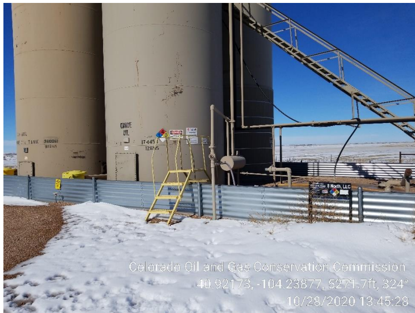
Photo 3 – West 17-34 Tank Battery – SE Crude Oil Tank missing Capacity Label
