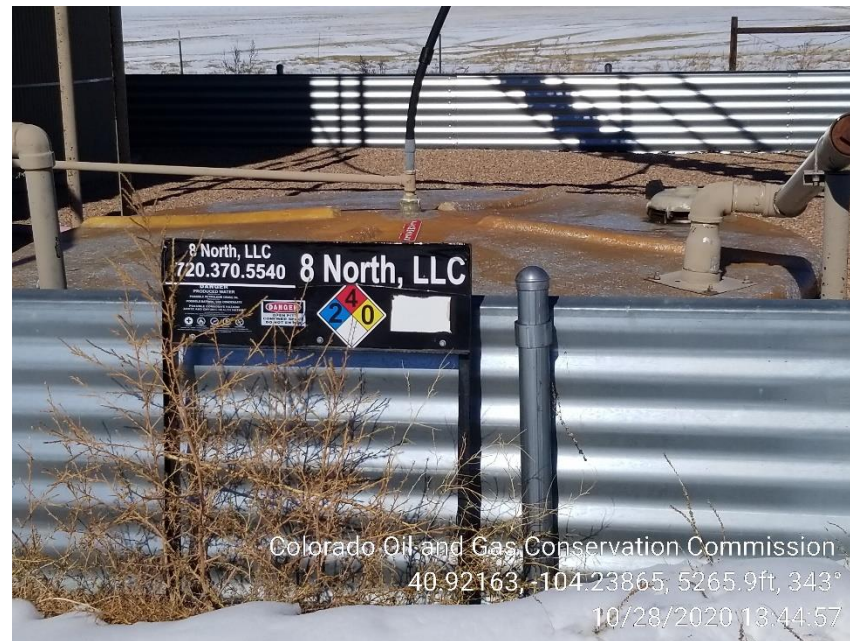
Photo 2 – Produced Water missing Capacity Label
