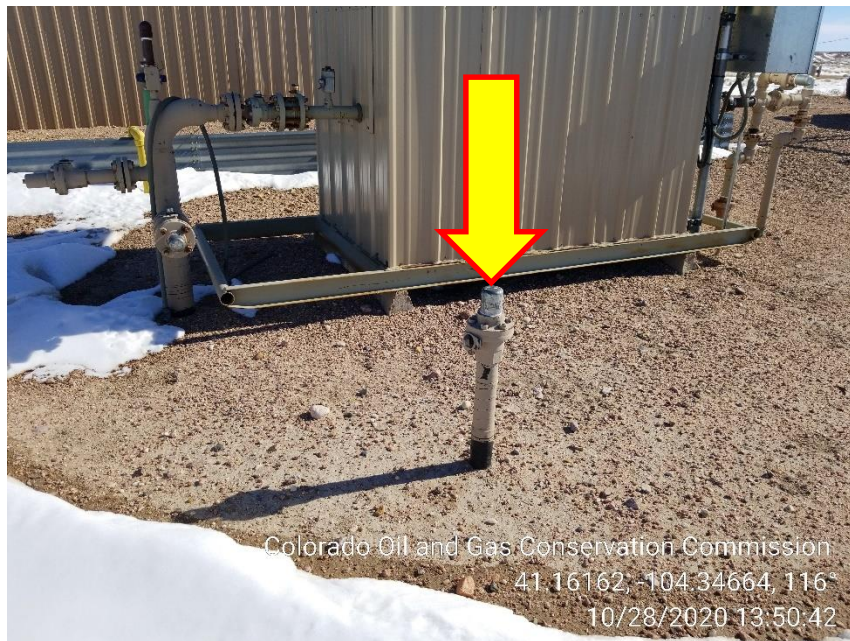
Photo 3 – East 17-99HZ Unmarked Riser at Gas Meter House
