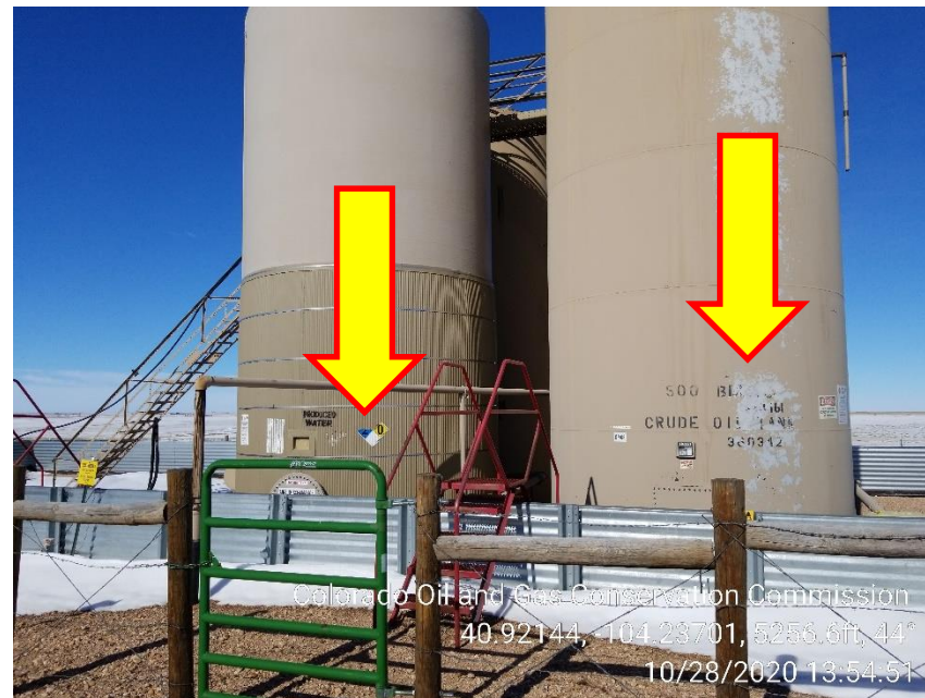
Photo 2 – Produced Water and Crude Oil Tanks missing NFPA Labels
