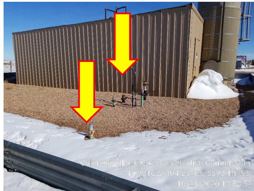
Photo 4 – East 17-99HZ Unmarked Riser at Heater Shed
