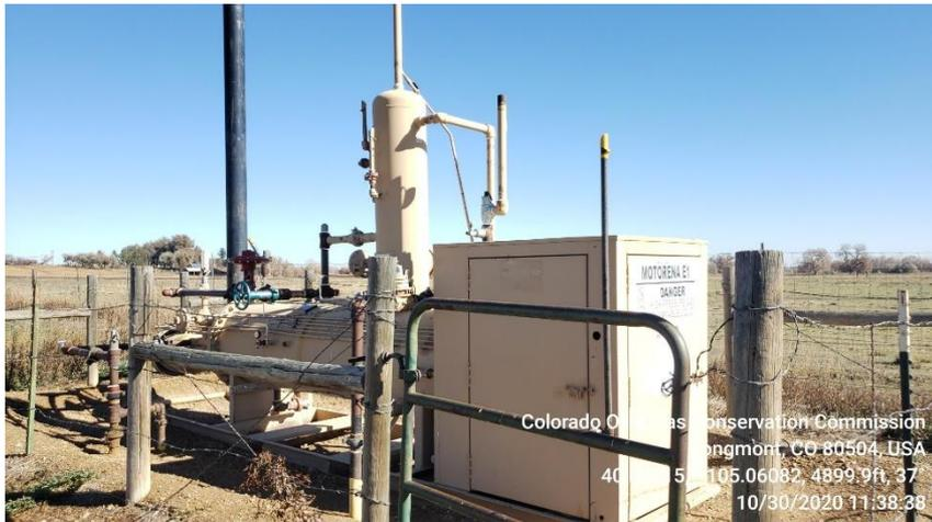
**Photo 5 Horizontal Heated Separator**
