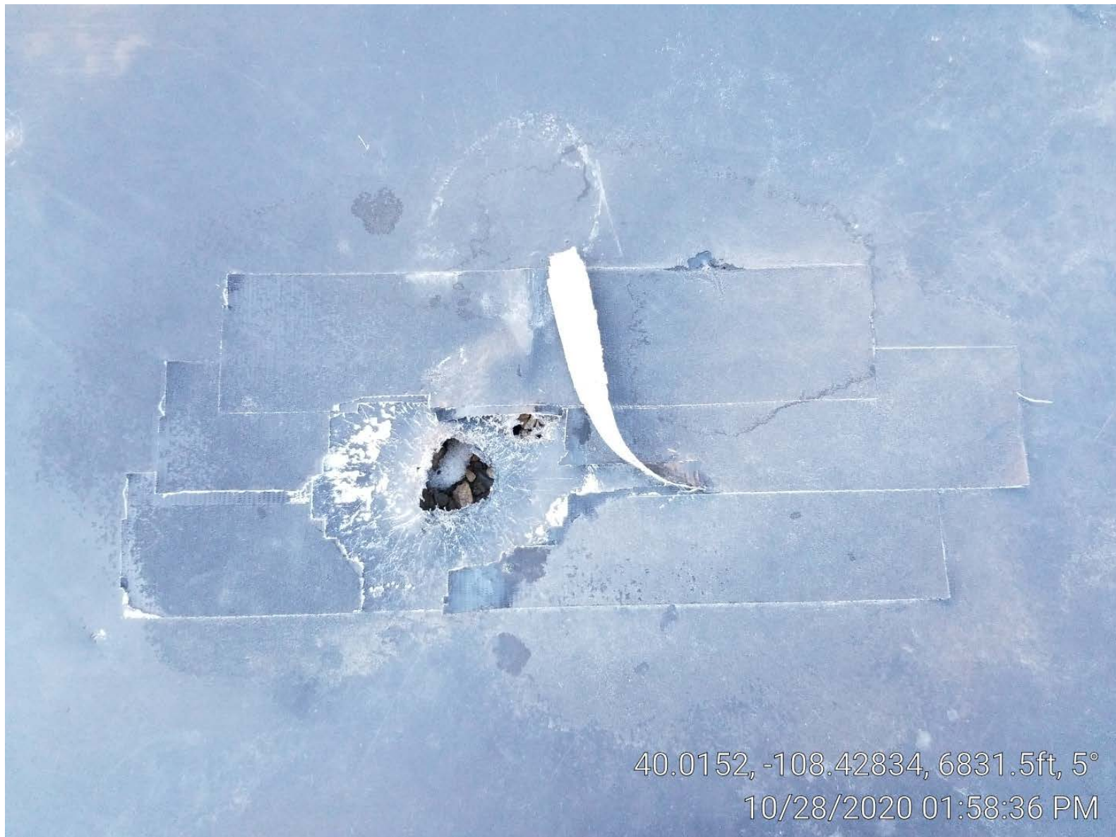
Photo 7. Hole in tank liner.
