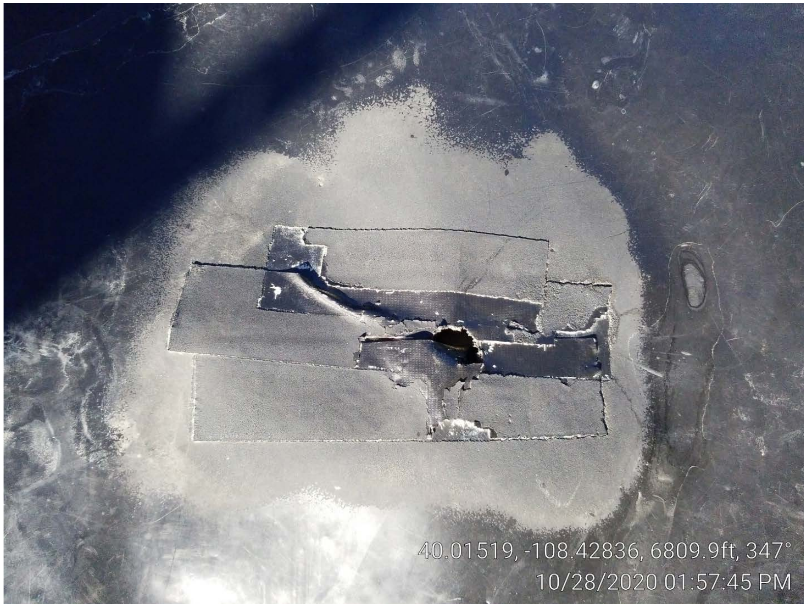
Photo 6. Hole in tank liner.
