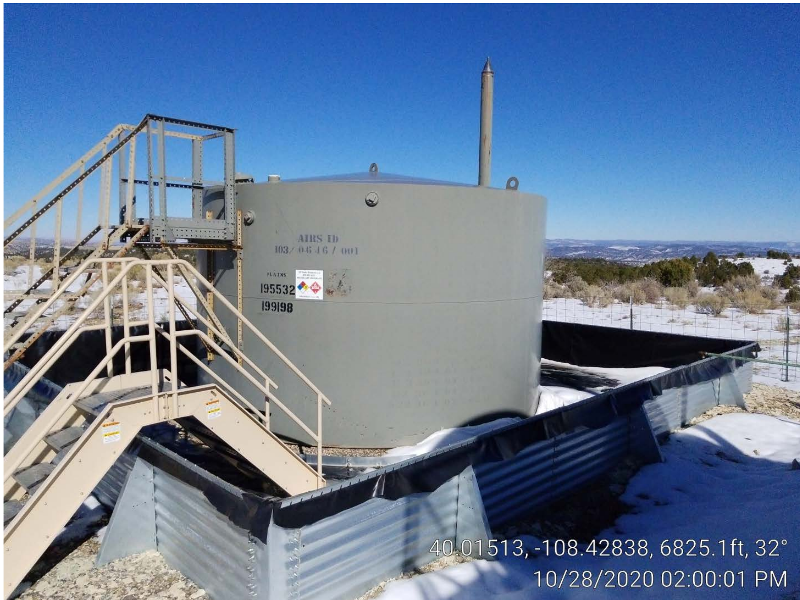
Photo 5. Tank with secondary container liner holes.
