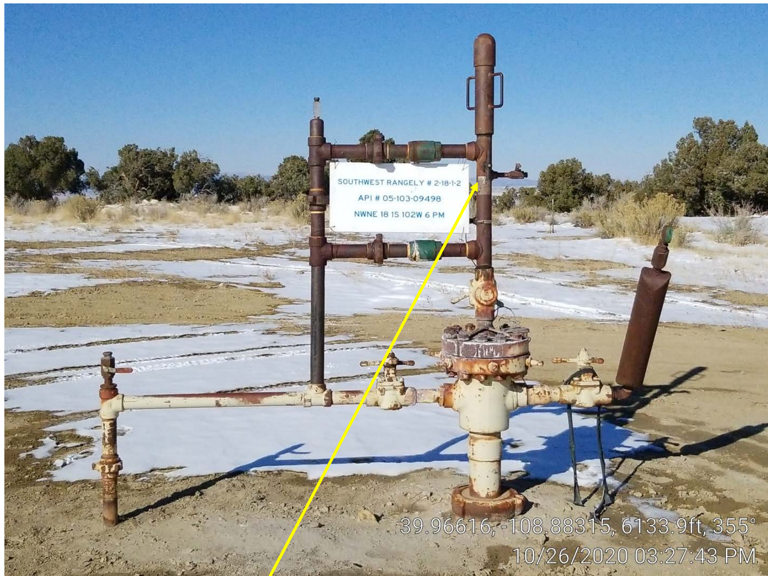
Photo 3. Well with gas leak.
